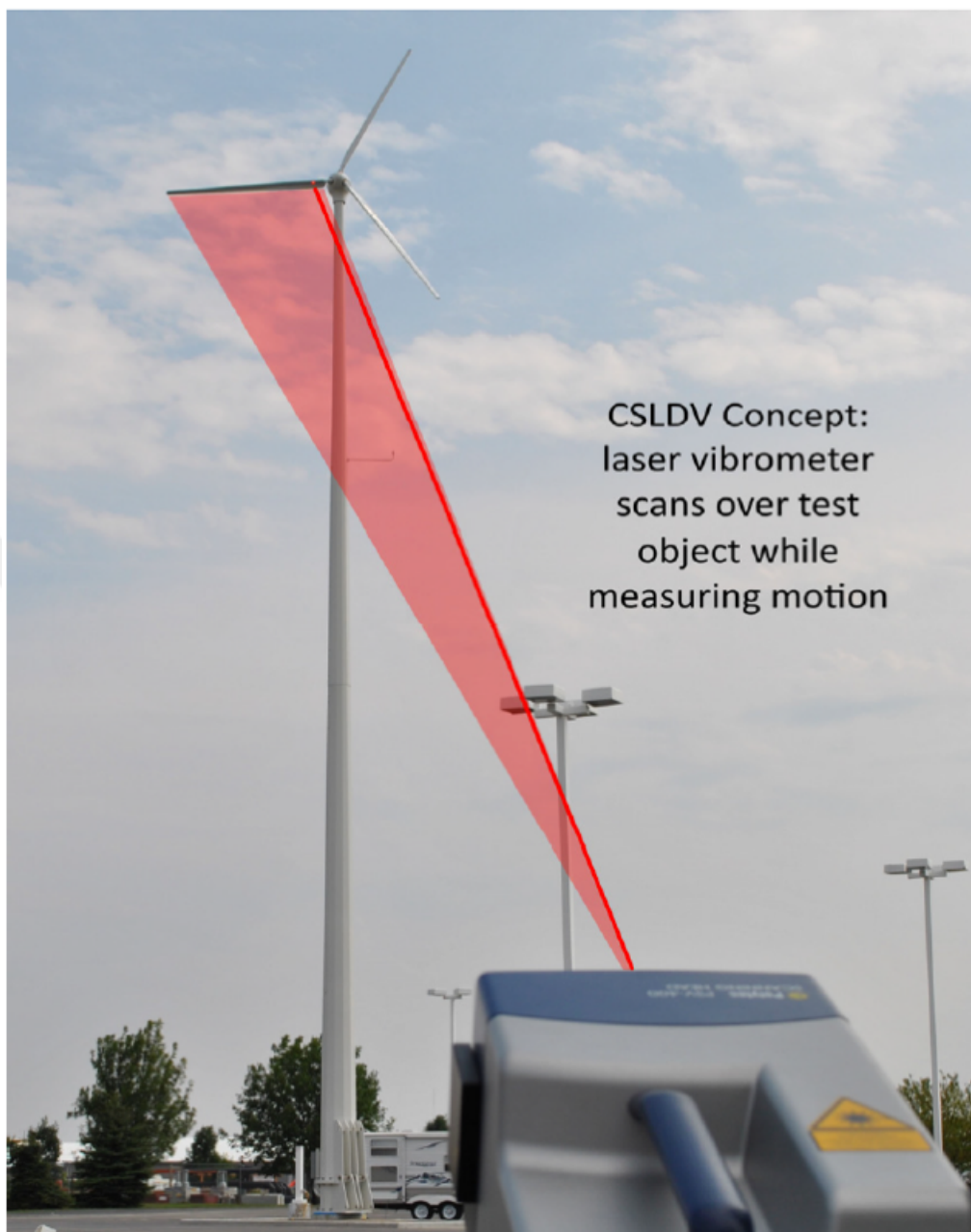
Figure 1.7. Continuous-scanning tests and short range laser measurements on wind turbines [23]
