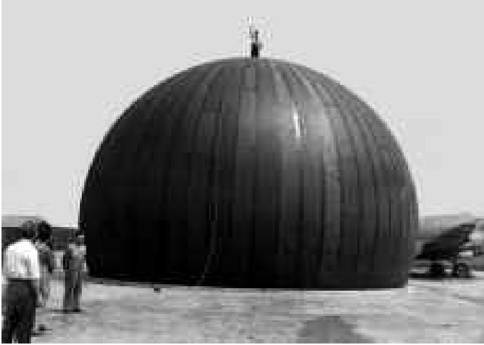
Şekil 3.20: Radar Dome, USA,1948,Walter Bird [Url-47]
