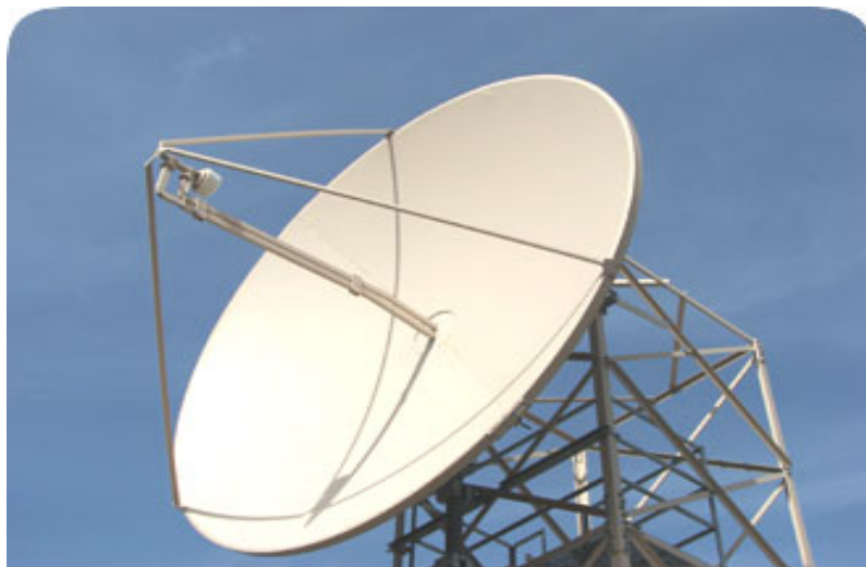
Figure 2.5: The Reflector (parabolic) antenna shapes
