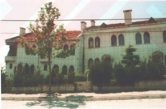
Figure 38: Tilted buildings in the southern part of Gürpınar.
