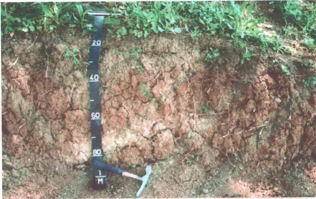
Figure 32: The clayey soil causes creep in the western part of Gürpınar.
