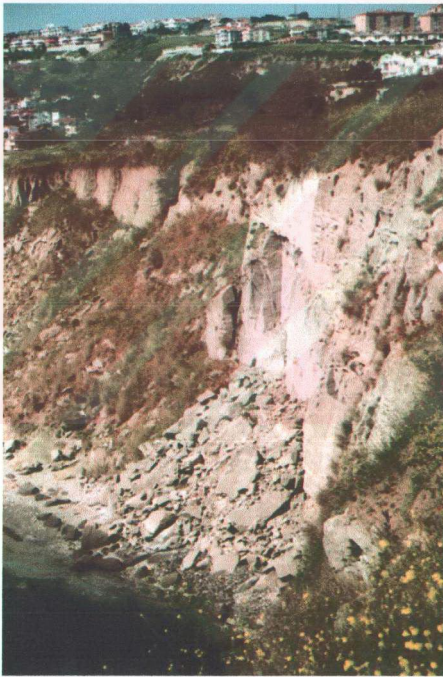
Figure 24: Current rock fall on the northeast coast of the Cape Mandabaşı.
