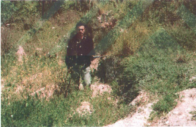
Figure 23: Concave scarp of a rotational slide in the southern part of Gürpınar.
