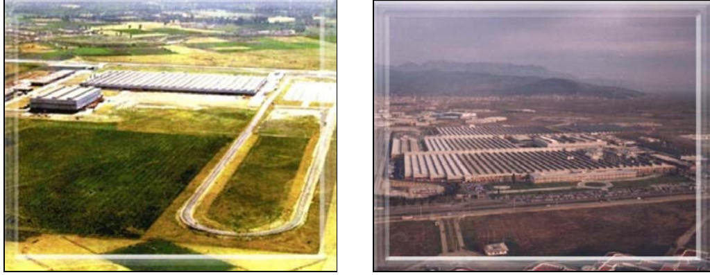
Figure 3.1. Tofaş Factory's view from above in the year 1970 and 2004
