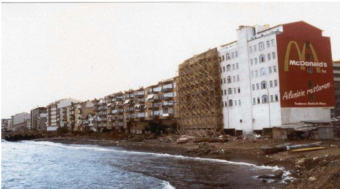
FIGURE 46: A CONSTRUCTION VIEW FROM TRABZON COASTS, NOT IN LINE WITH THE LEGISLATION
