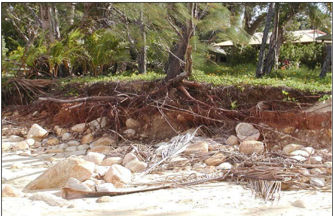
FIGURE 27: ROCK AND SOIL FILLL MATERIAL ON THE ESPLANADE EXPOSED BY DUNE EROSION
