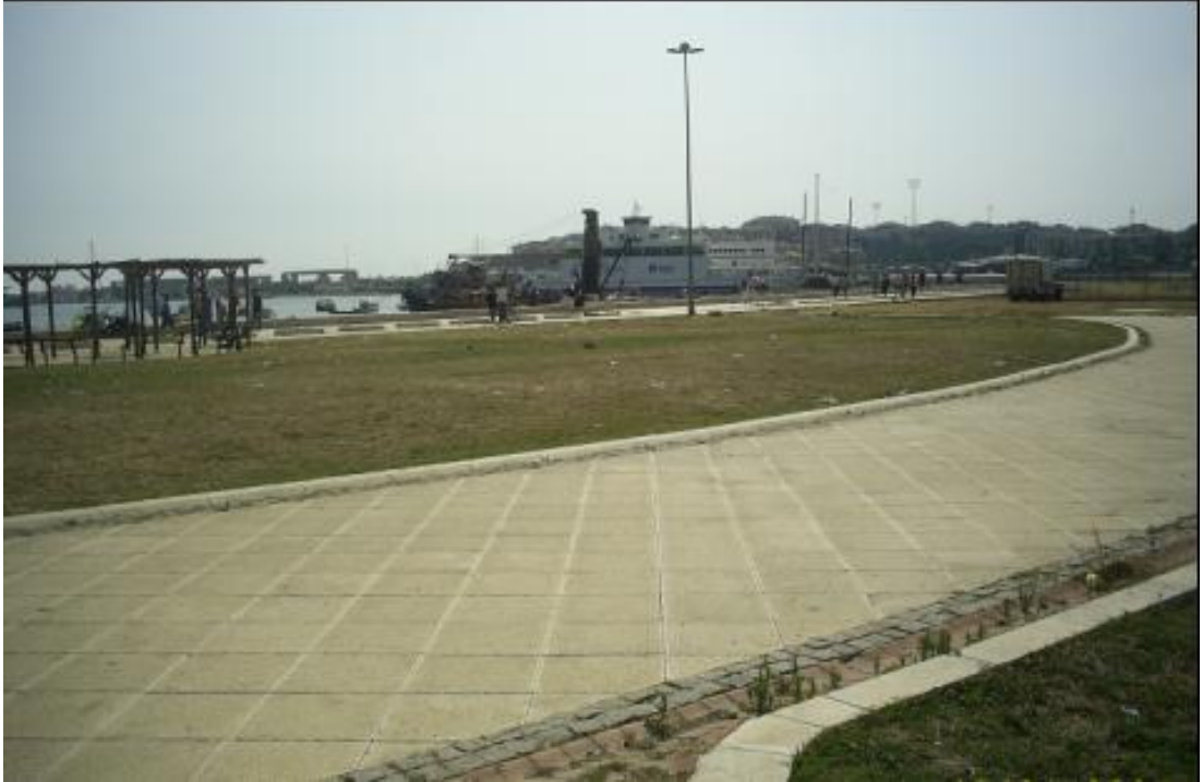
FIGURE 48: COASTAL FILLING AREA AND PORT OF PENDİK
