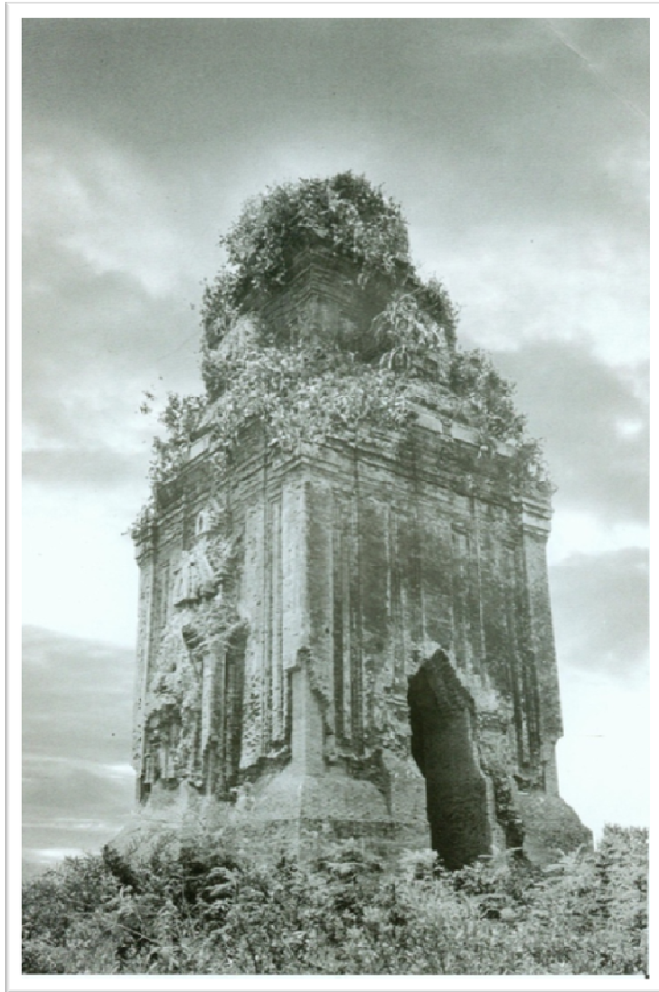
Figure 3 – Phu Loc Tower (Phuoc Loc tower) was built in 12 th century on top of a hill in Phuoc Loc village, Nhon Loc commune, An Nhon district, Binh Dinh province. The tower is 29m high with a square base of 9.7m x 9.7m. As it lies on a hill 76m high, it can be seen by visitor from a far distance. This tower is also known as Cao Mien tower and called by the French as golden tower (Tour d' Or) , from the Heritage of Cham Culture collection of Nguyen Van Ku.
