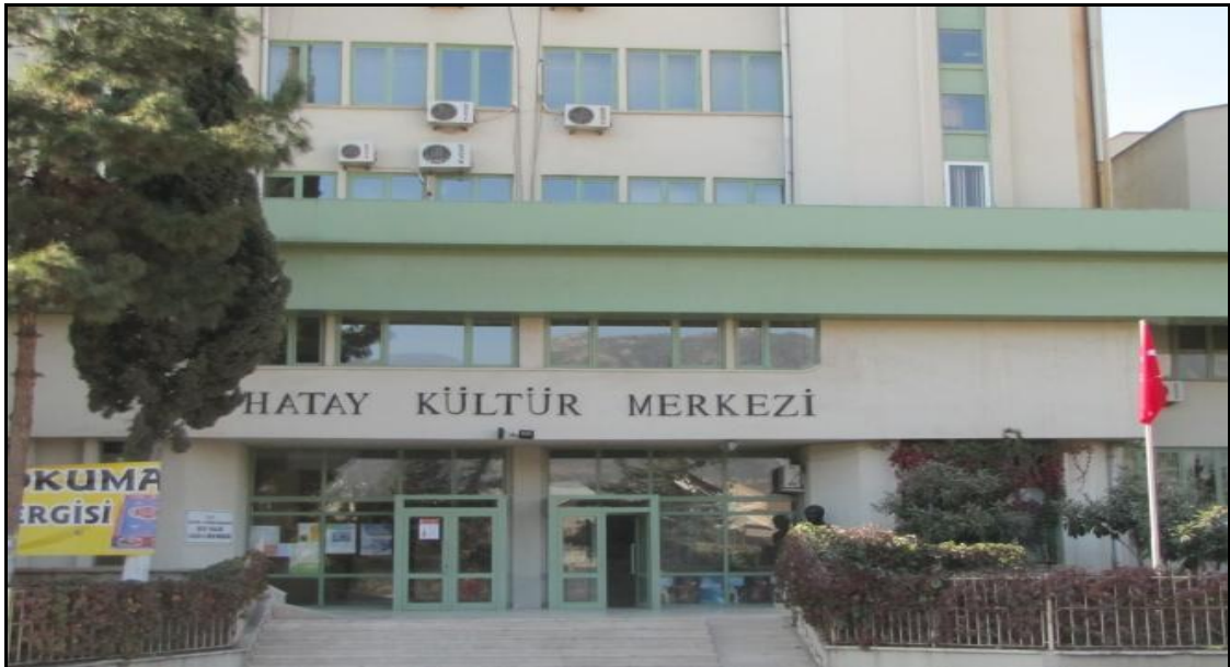
Figure 6.25. Cultural building a place various cultural activities in Hatay
