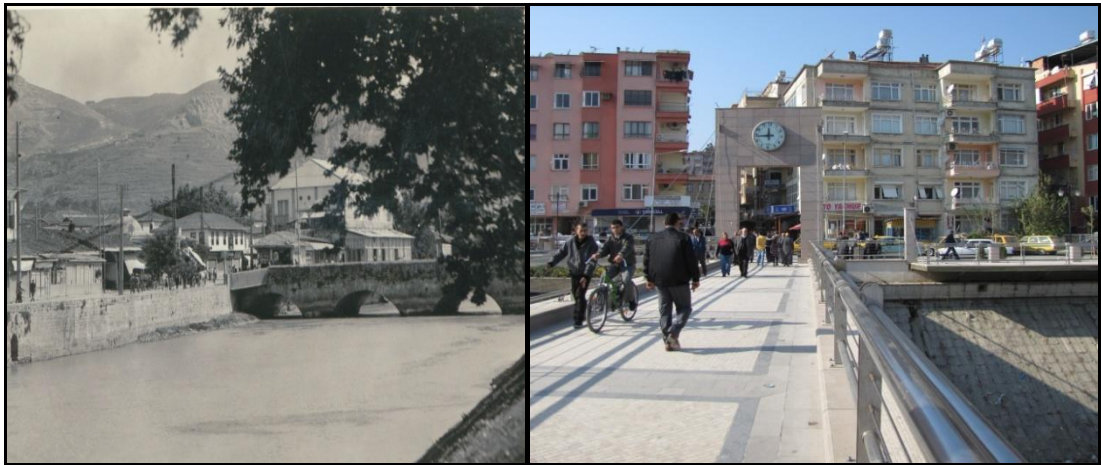
Figure 6.15. Collapsed bridge of Rome and the concrete bridge at present
