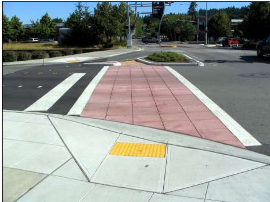
Figure 27. A sample of a secure slope – Washington – U.S. ( www.pedbikeimages.org / Dan Burder)
