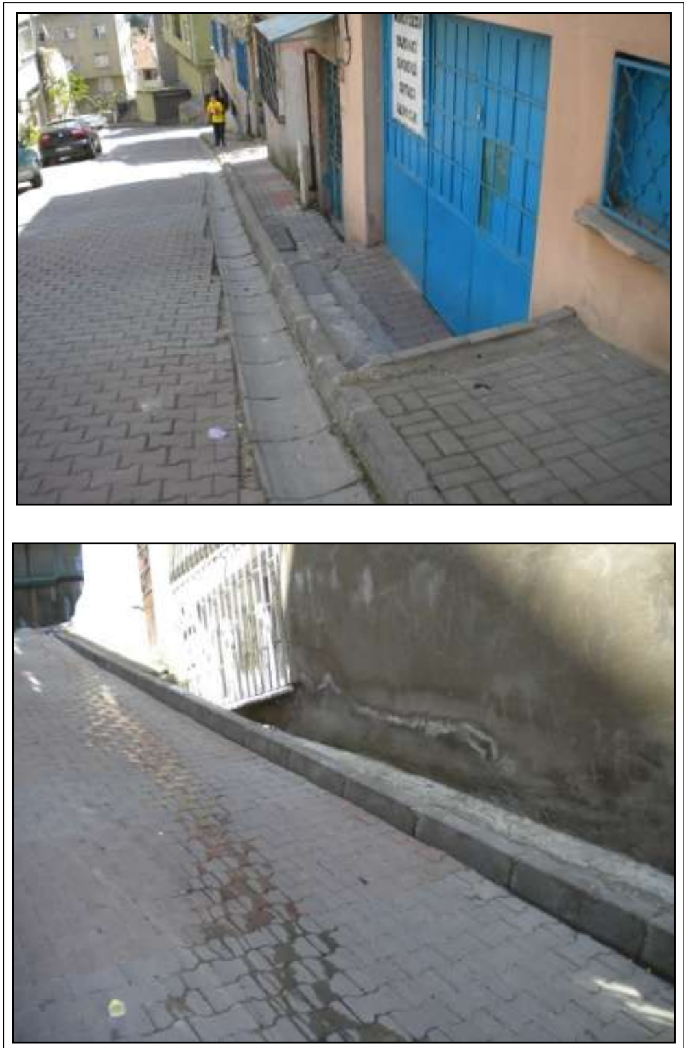
Figure 51. Slope exceeds 8%
