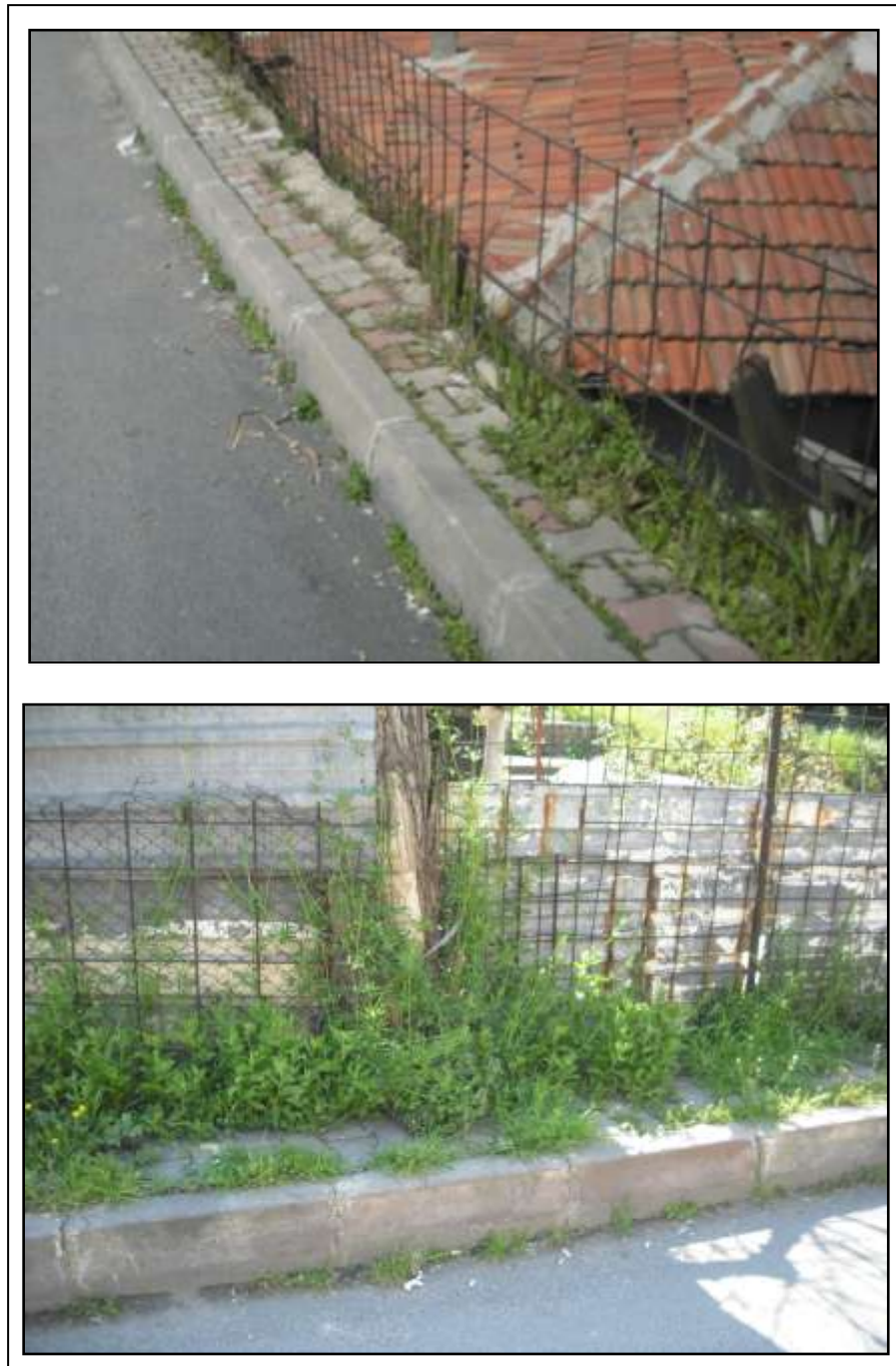
Figure 42. Pavement segments which have less than 50 cm width
