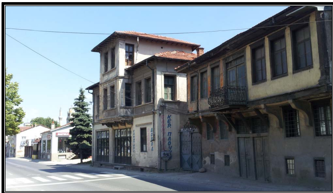
The existing buildings on May 1st Avenue (Булевар 1-ви) next to the Telegram House of Manastir where Şemsi Paşa was killed. (Photo: Hakan Özdemir, 2012)
