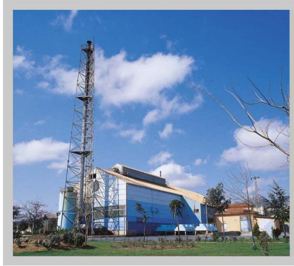
Figure 1.17 ISTAC Co. Ltd. Medical Waste Incineration Plant [ISTAC, 2011]
