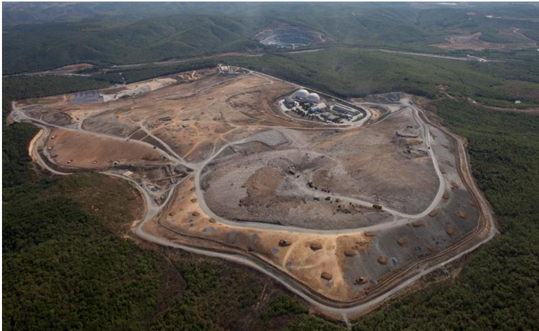
Figure 1.8. Sanitary Landfill Site [64].
