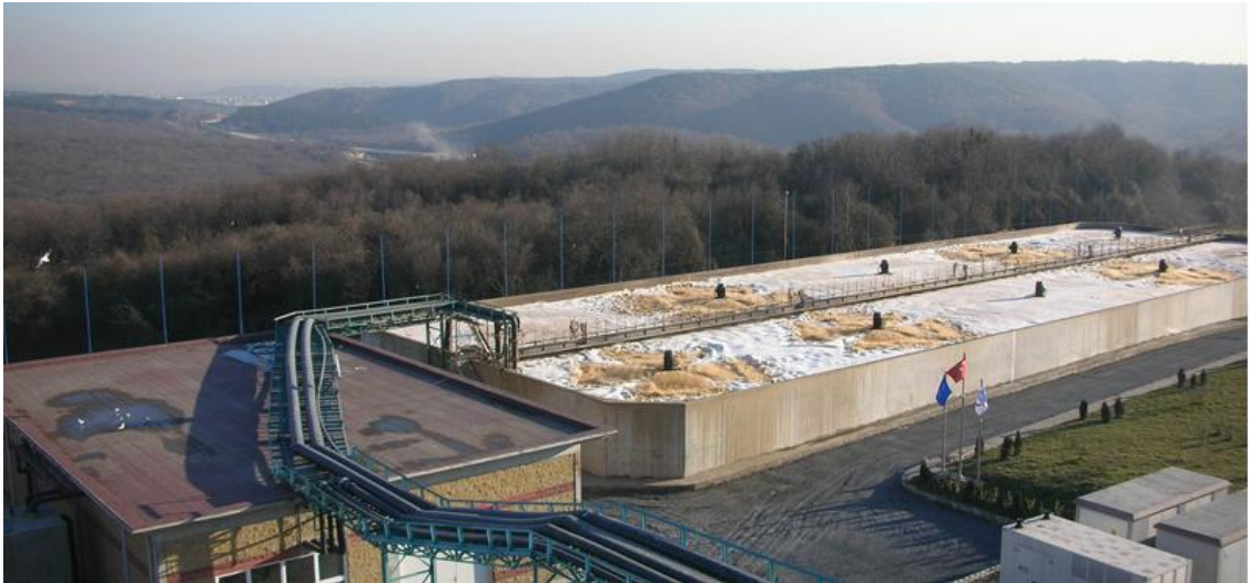
Figure 1.10. A Wastewater Treatment Plant [64].
