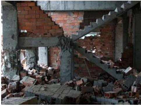
(a) Damage to “short columns” under platform
