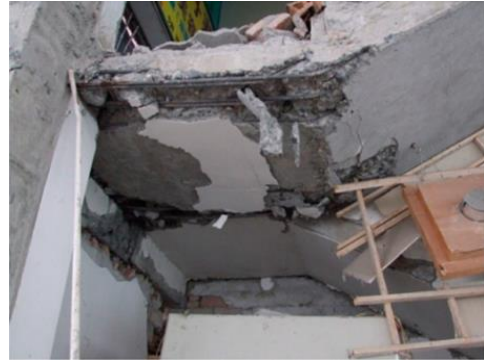
(b) Damage to horizontal slab and landing beam
