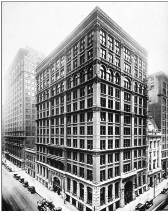
Figure 2.1 : Home Insurance Building
