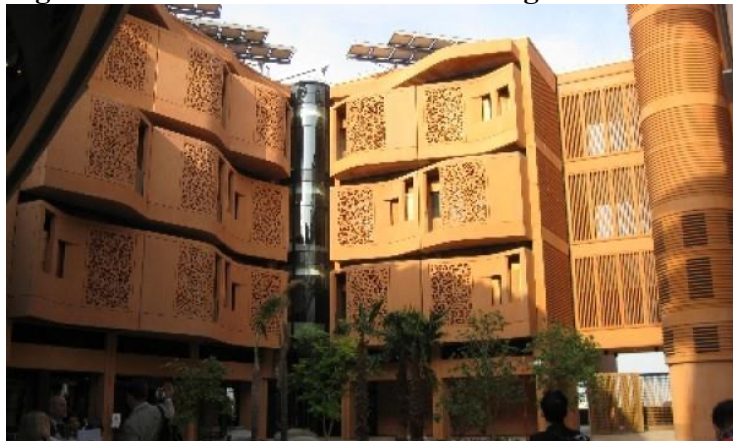
Figure 3.8: Masdar Institute's buildings
