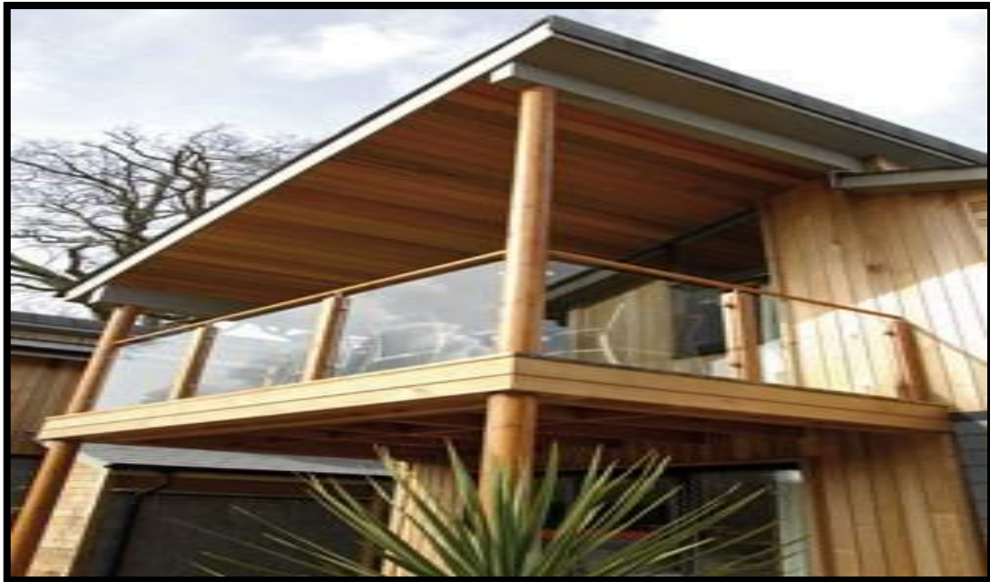
Figure 2.51: Prefabricated wood frame building in UK
