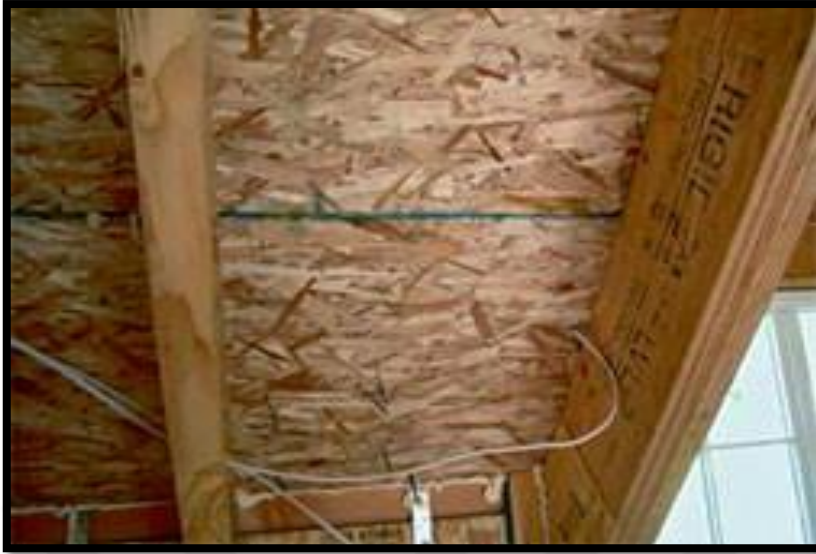
Figure 2.42: Example of SIPs used for roof panels
