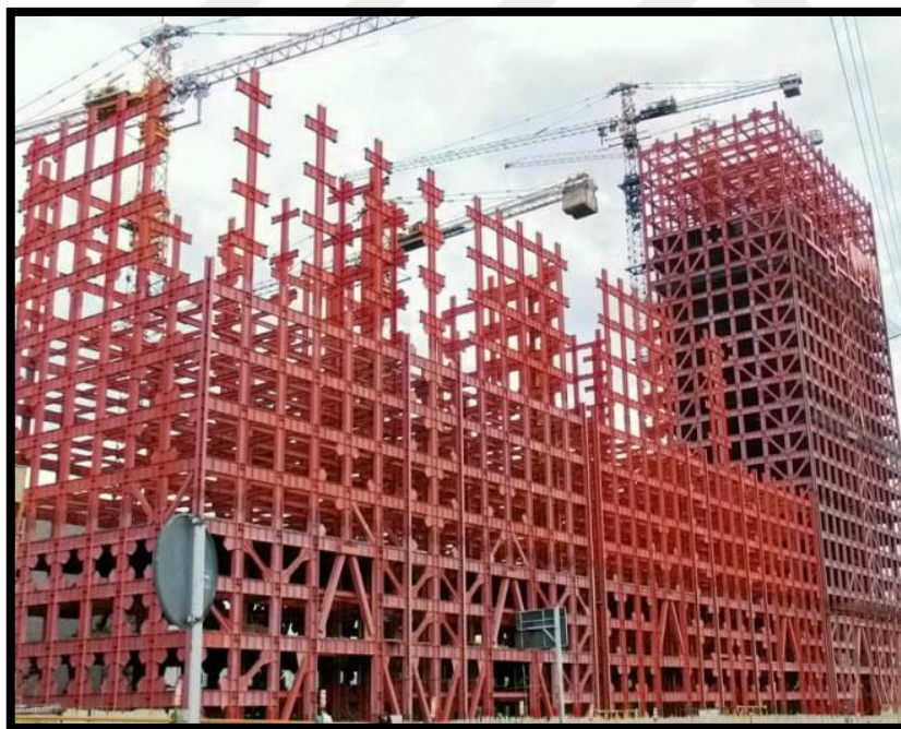
Figure 2.52: Steel frame system in Iran
