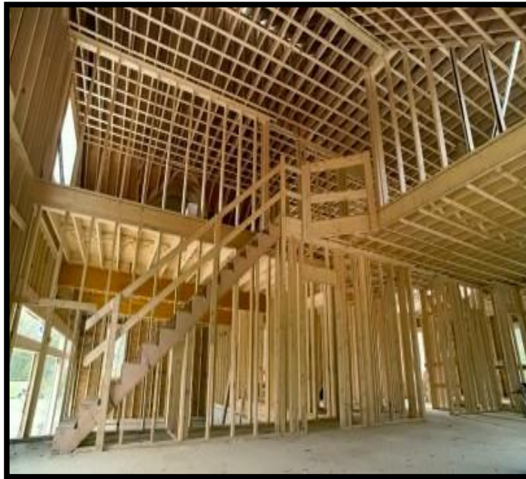
Figure 2.25: Example of Platform wood frame systems
