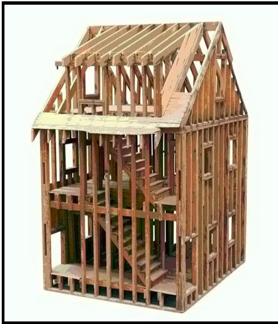
Figure 2.27: Balloon wood frame system
