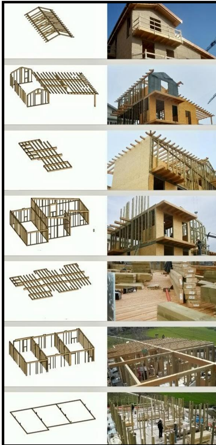
Figure 2.26: Platform wood frame systems process
