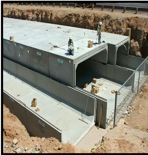
Figure 2.47: Cells system in construction
