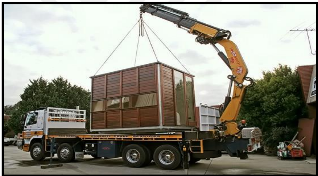
Figure 3.3: Prefabricated building being transported by vehicle
