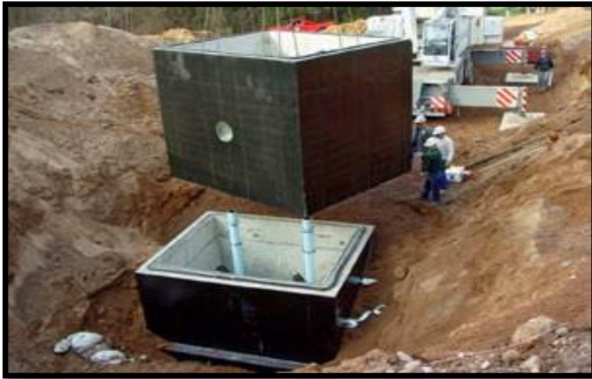
Figure 2.12: Completed prefabricated chamber
