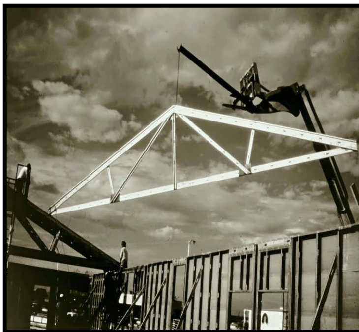
Figure 2.16: Installing roof trusses
