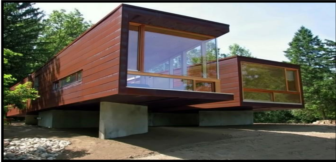
Figure 2.15: Modular prefabricated building
