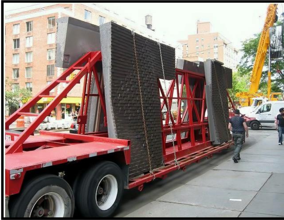
Figure 3.4: Prefabricated components being transported by vehicle
