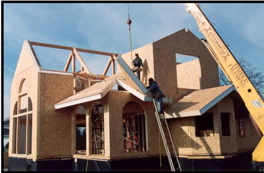
Figure 2.40: Structural insulated panel in building construction
