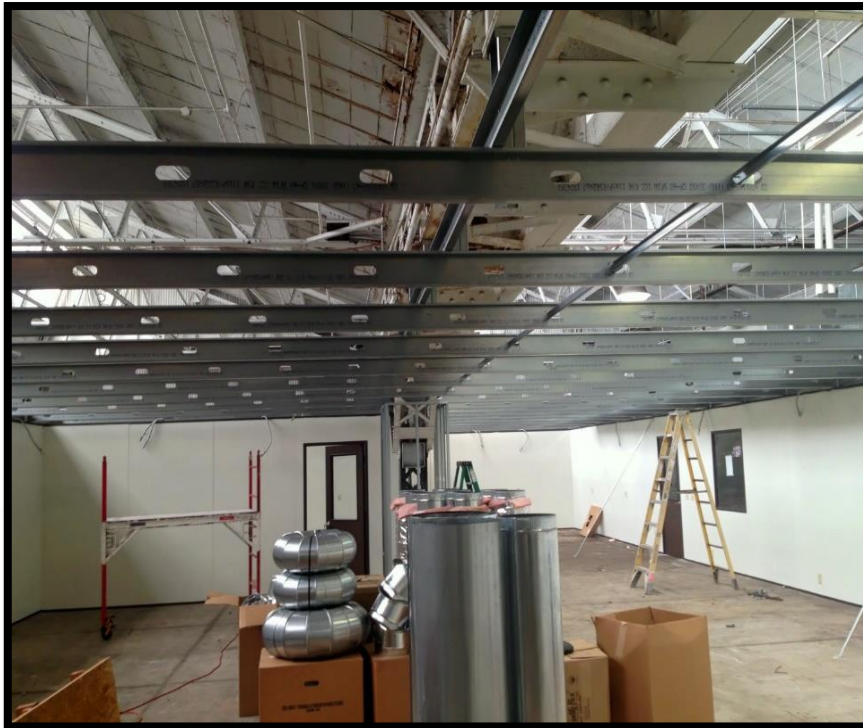
Figure 3.1: Installation of floor joists in an enclosed environment
