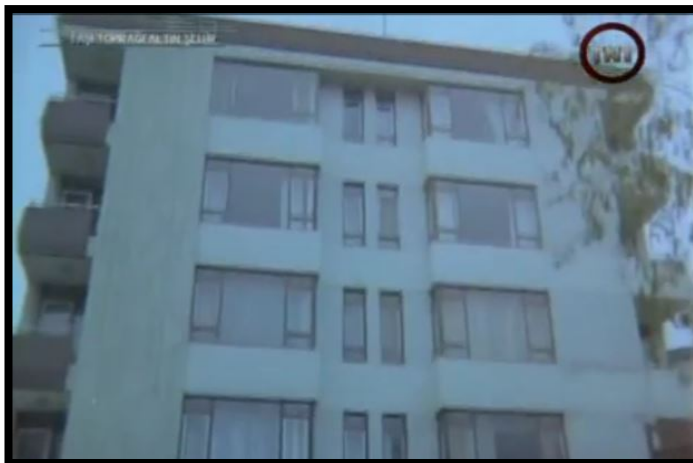
Figure.42: Fatma Works in a Modern Apartment Block
