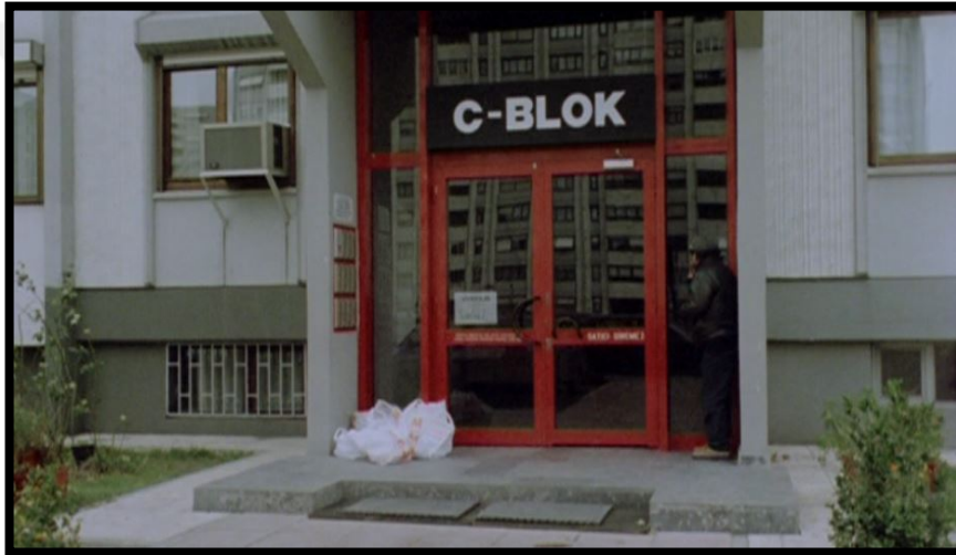
Figure.45: Entrance door of Block C
