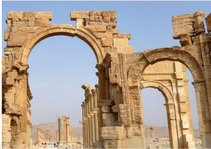
Figure 3.13: Slippage between the Blocks in Arch in Syria
