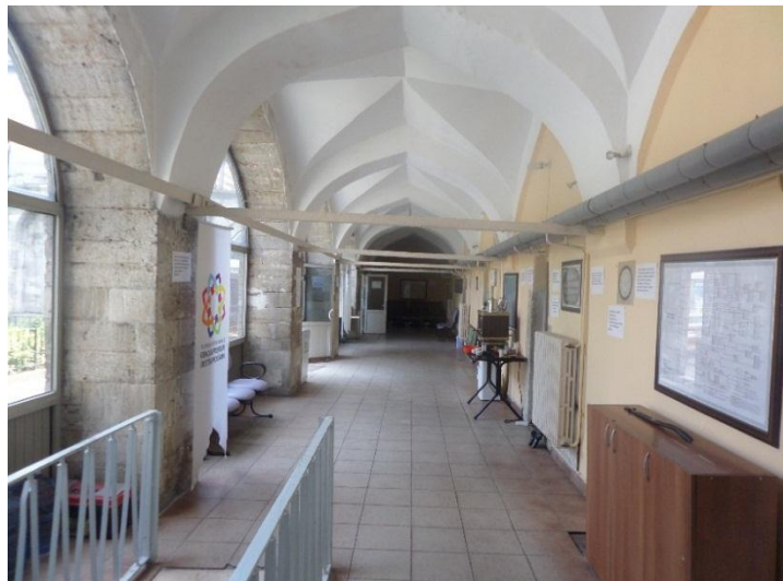
Figure 5.51: The Addition of Pipes and Electric Wires in Arcade
