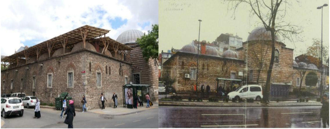
Figure 6.3: The Lead of Domes 1. After Removal 2. Before Removal
