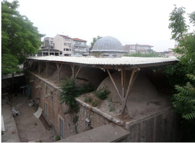
Figure 3.44: The Remove of Lead of Domes
