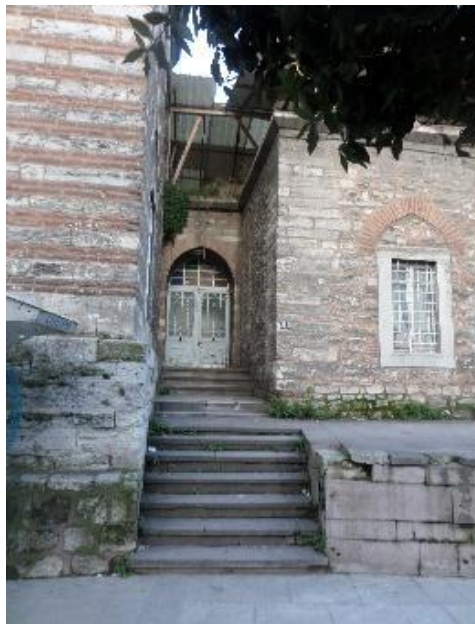
Figure 6.2: The Right Side Entrance of the Madrasa
