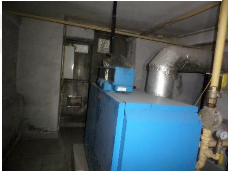
Figure 4.28: First Basement Room
