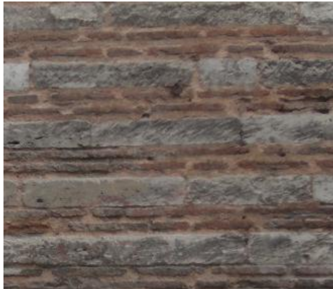
Figure 4.36: Bricks on the Southern Facade
