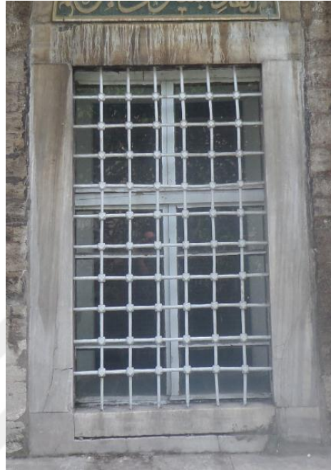
Figure 5.27: Window of Classroom (G5G6F5F6)
