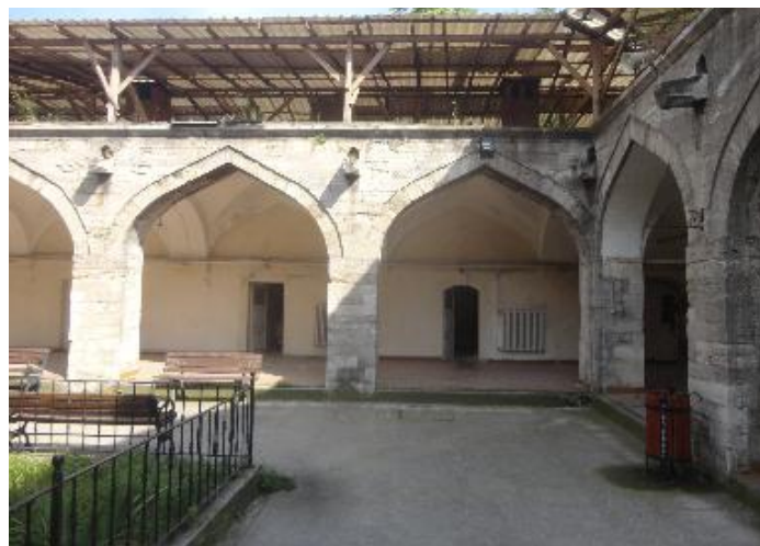
Figure 4.41: Archs of Arcade
