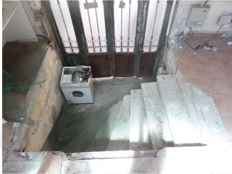
Figure 5.52: The Addition of New Staircase
