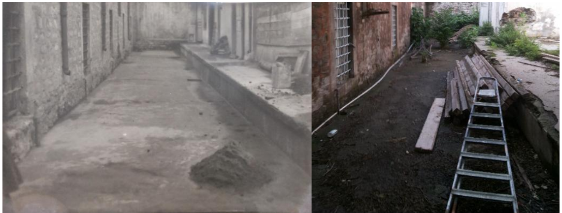
Figure 5.45: Intervention of Side Courtyard
