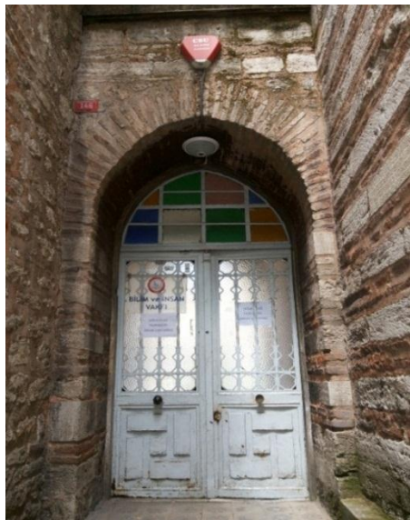
Figure 4.43: Arch of the Exterior Entrance
