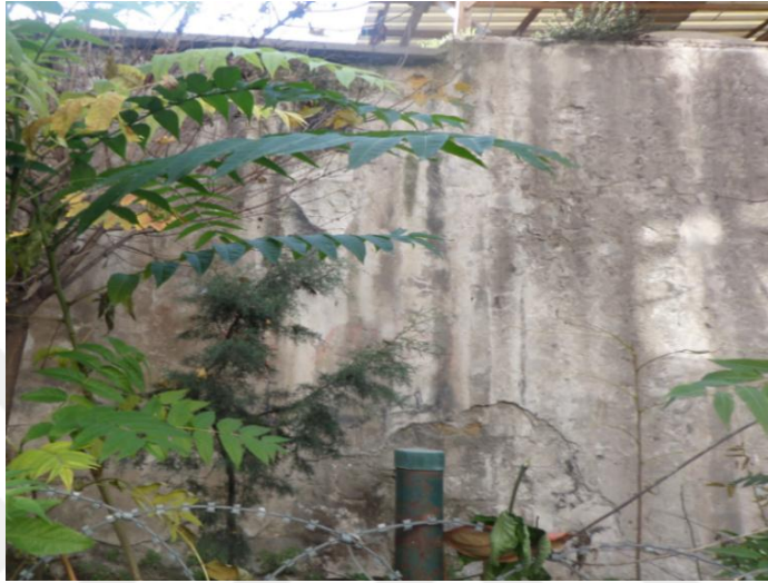
Figure 4.35: Lime Based Plaster on Northeastern Facade
