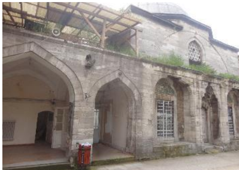
Figure 4.39: Façade of Classroom
