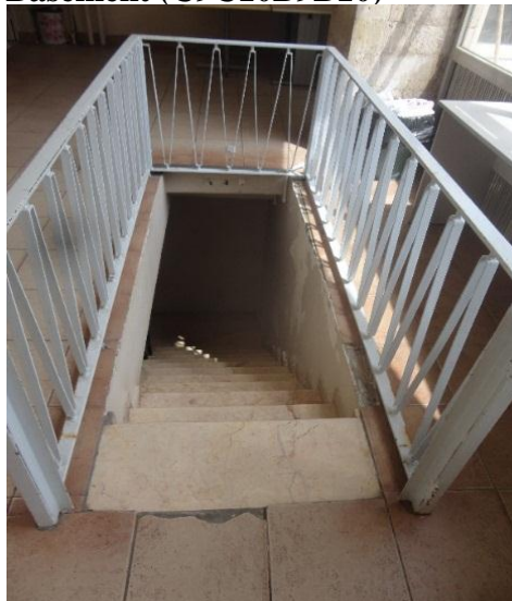
Figure 5.43: the Stairs of Basement (C9C10B9B10)
