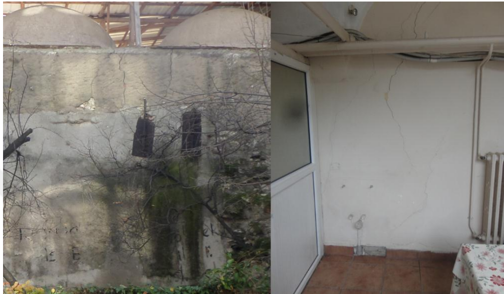
2. Interior Face of wall
