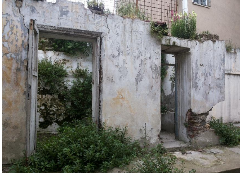
Figure 5.47: Addition of Toilets of Side Courtyard
