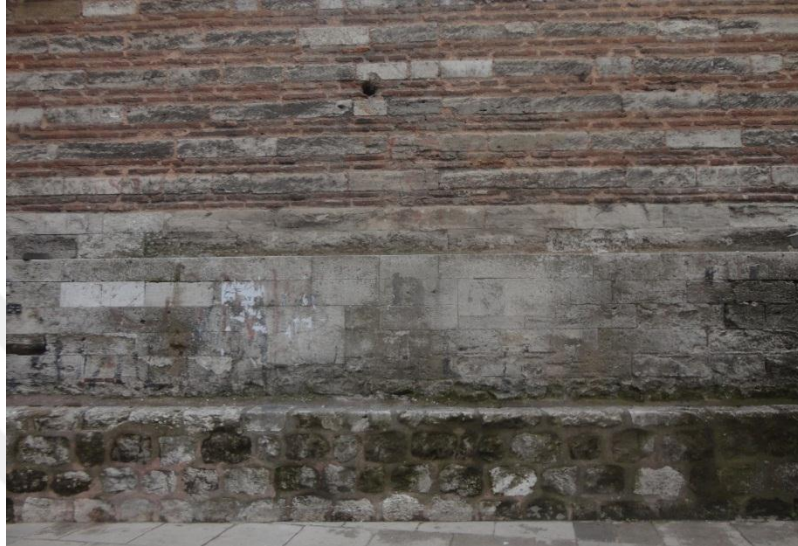
Figure 4.38: Center Part of Southern Facade
