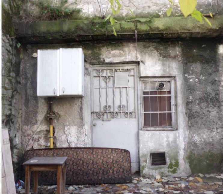
Figure 5.54: The Addition of Door (A10A11)
