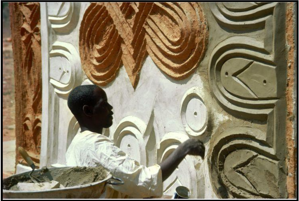
Figure 3.1: Making of some patterns on wall surface
