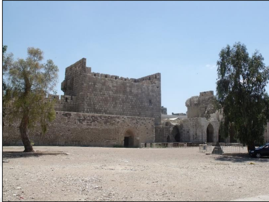
Figure 4.52: Neglected Space inside the Old Castle
