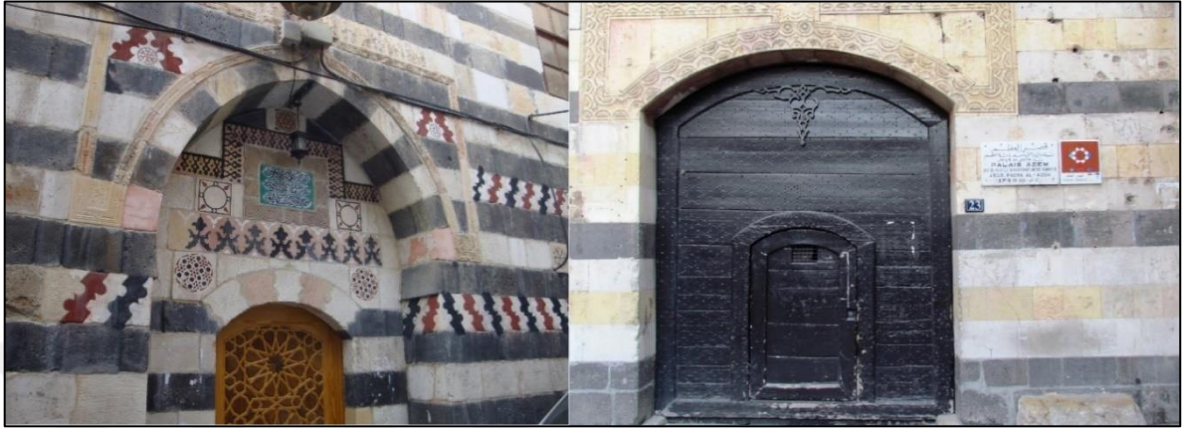
Figure 4.10: Entrance of House near Bab Al-Jabia (Left Picture) and Al-Azem Palace Entrance (Right Picture)
