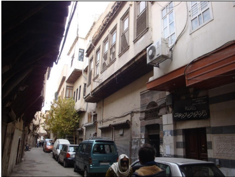
Figure 4.44: A House with Small Wooden Covered Windows
