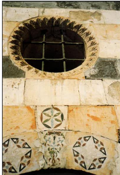
Figure 4.47: Circular Opening in Al-Sibaei House
