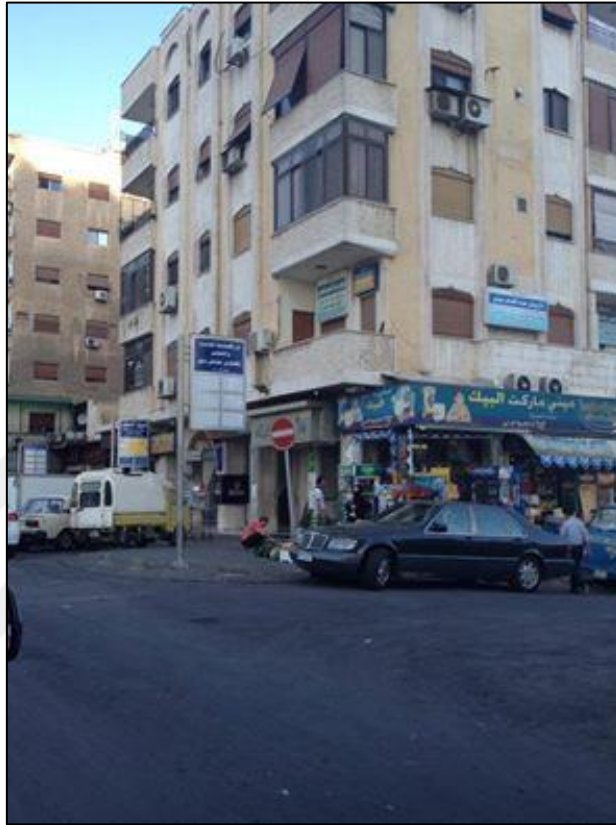
Figure 4.118: Large Fixed Windows Covered with Aluminum Shutters
