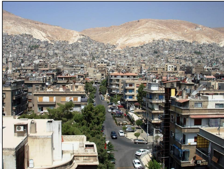
Figure 4.82: General View of Part of Modern Damascus
