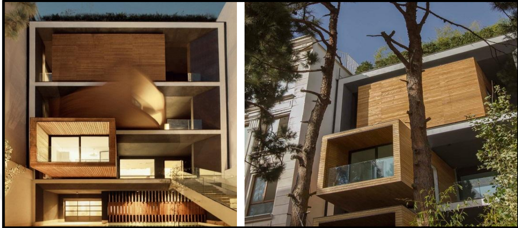
Figure 4.6: Sharifi-Ha house narrow façade and movable boxes
