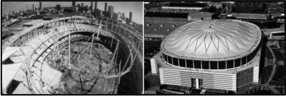
Figure 2.11: Georgia Dome, Atlanta, 1992
