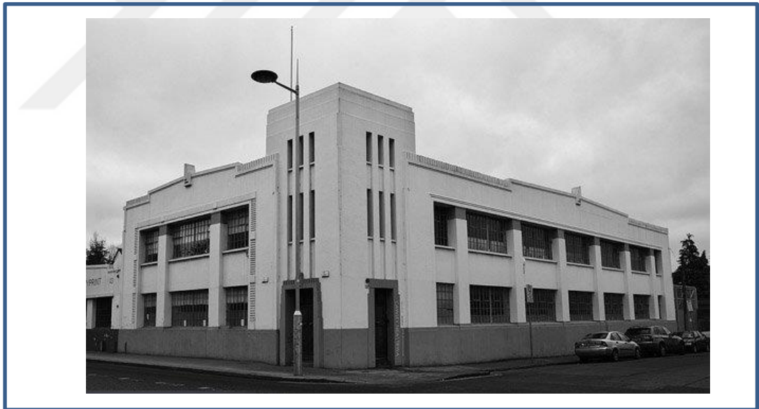
Figure 3.2 Kodak House Exterior View
