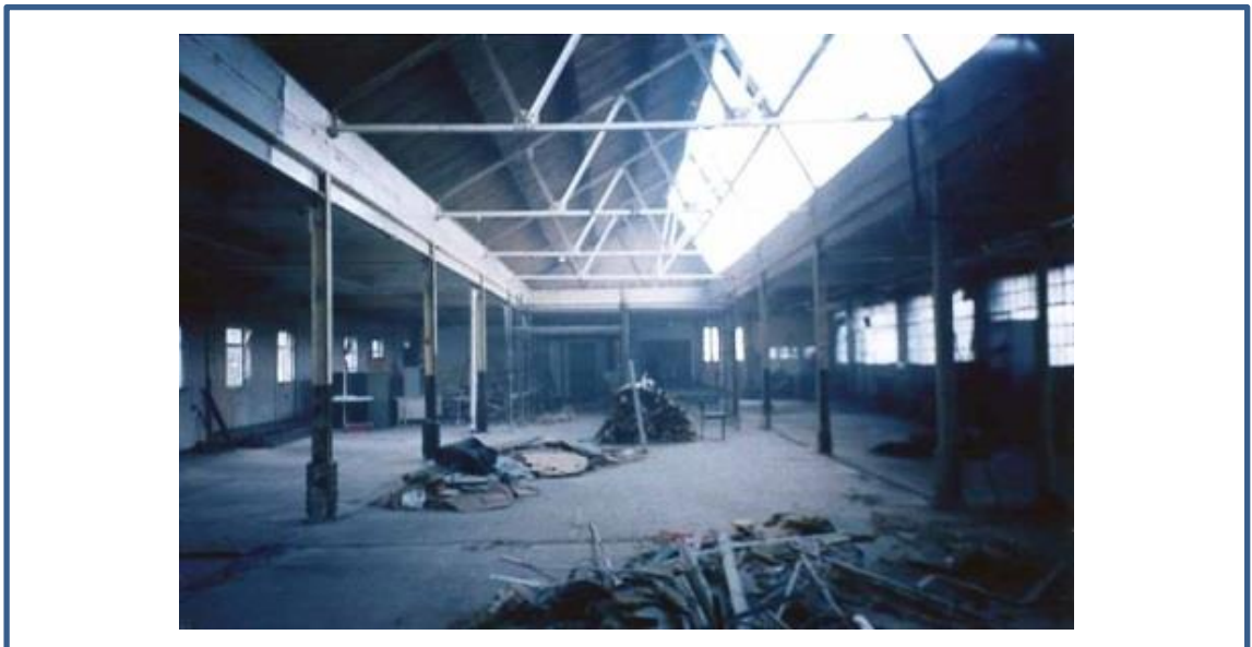
Figure3.3: Old Interior situation of the Kodak House
