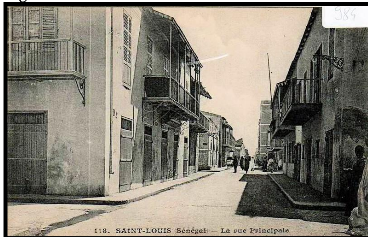
Figure 3.9: Civil colonial architecture
