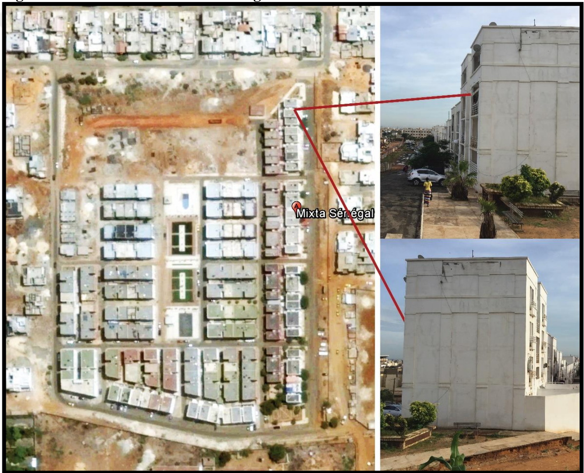
Figure 3.13: Pictures of Mixta building
