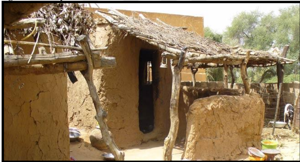
Figure 3.6: Clay construction and wooden structural elements
