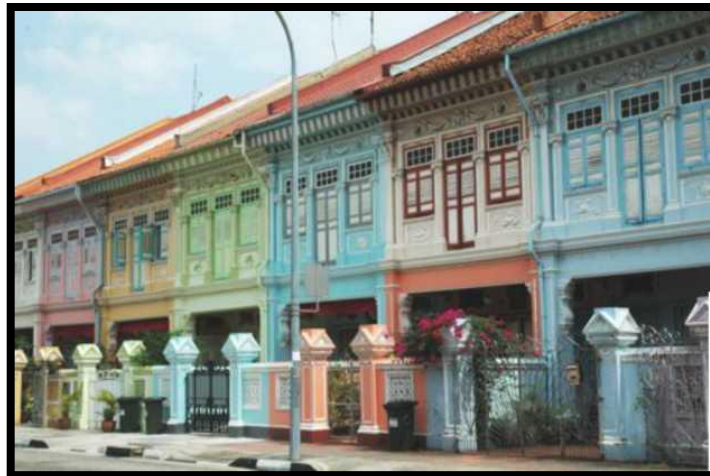
Figure 5.15: Traditional Shop Houses with wooden louvers
