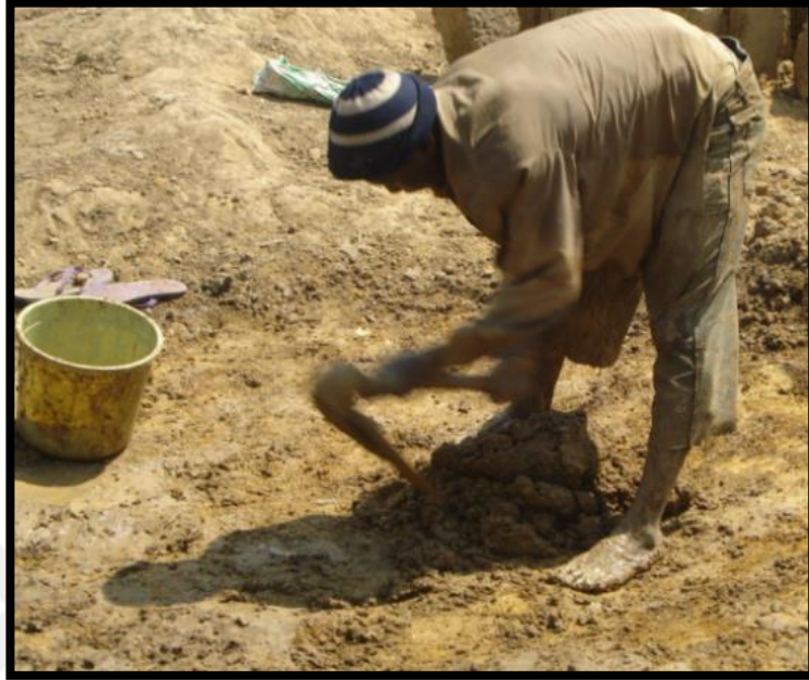
Figure 0.1: Mud for wall construction
