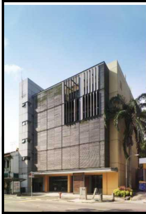
Figure 5.14: Exterior with bamboo louvers
