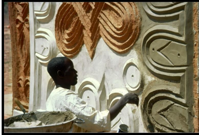
Figure 0.7: Cutting through wet cement
