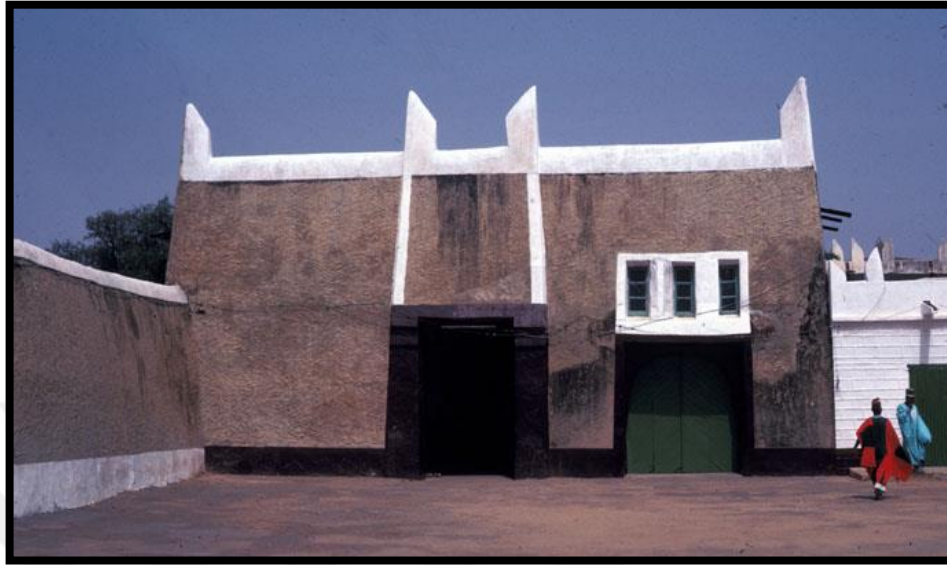
Figure 4.3: Gidan rumfa mud architecture
