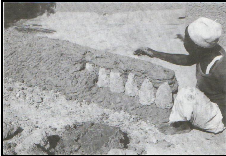
Figure 0.4: A man constructing the foundation of a wall
