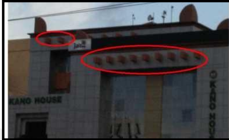
Figure 5.3: Gutter for rain passage
