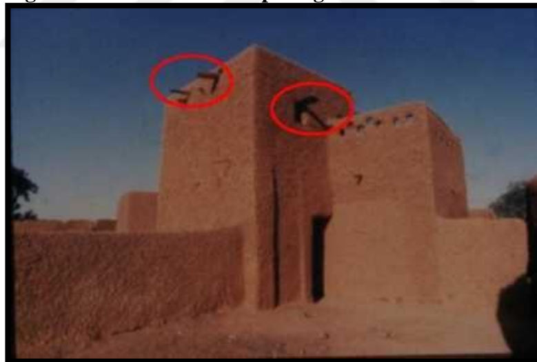
Figure 5.2: Gutter for rain passage
