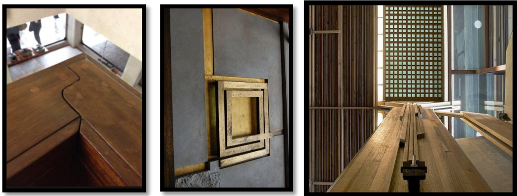
Figure 3.5: Carlo Scarpa Wood Joints; a) Wooden railing corner joint; b) Olivetti Showroom, Venice, Italy, 1957-58
