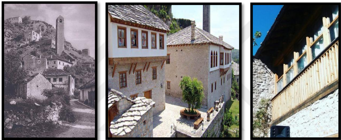
Figure 2.3: Houses of the City of Pocitelj
