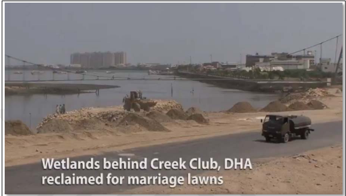
Figure 3.19: DHA Land reclamation behind Creek club at Clifton
