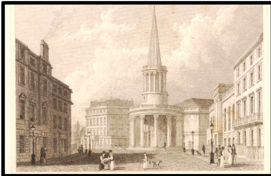
Figure 4.29: View of the east side of Langham Place, Regent Street, with the church in the centre, 1825
