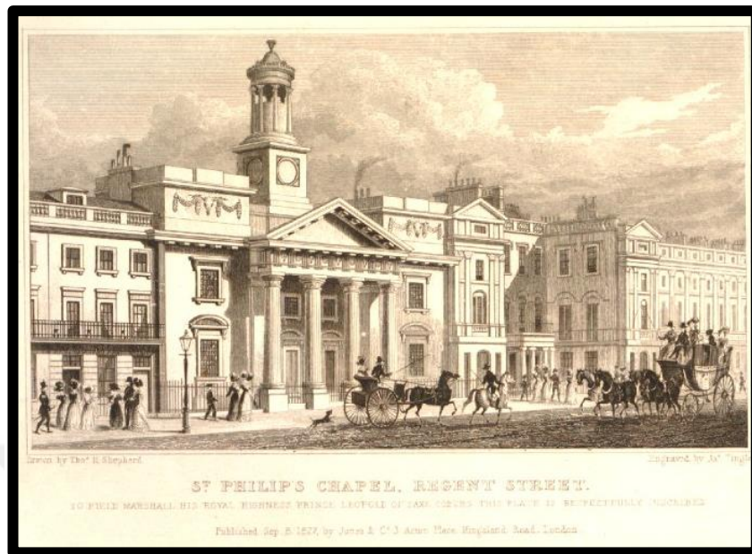
Figure 4.22: St Philip's Chapel, Regent Street, 1827
