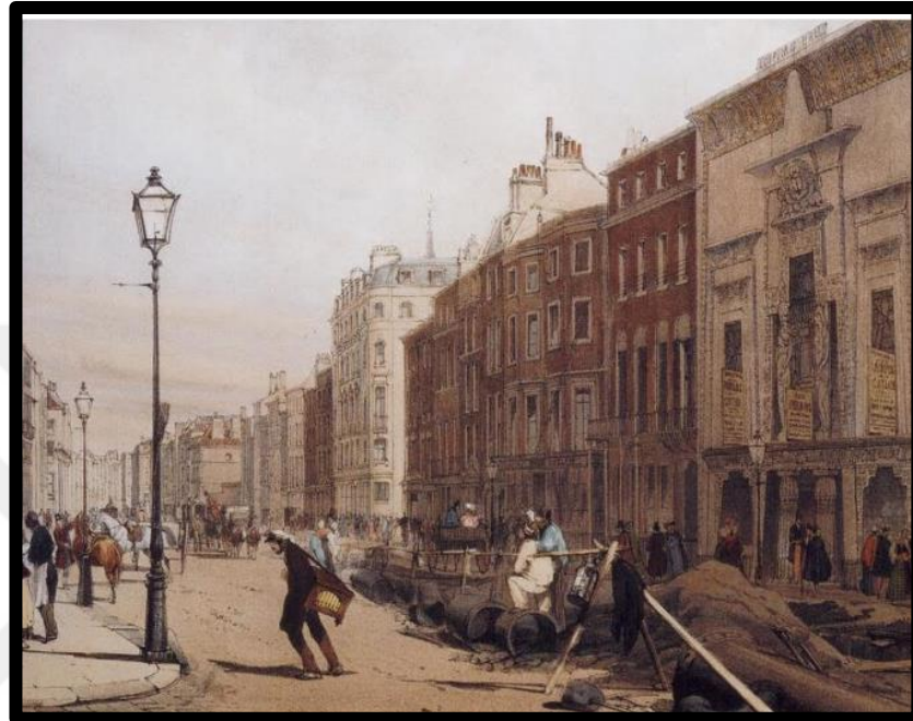
Figure 4.40: Sewer system being installed in Piccadilly (intersection between the Quadrant and Lower Regent Street)
