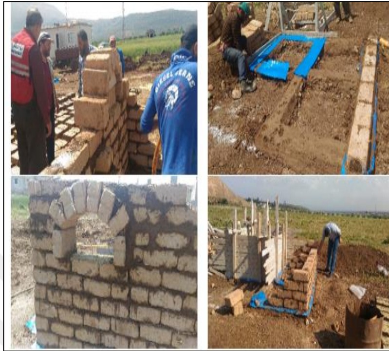
Figure 5.14: Mud Construction Training By QRC
