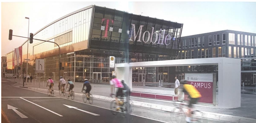
Figure 3.15: T-Mobile Headquarters in Bonn, Germany
