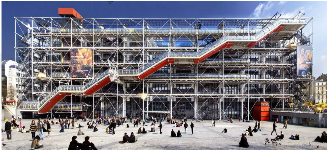
Figure 2.2: The Centre Pompidou
