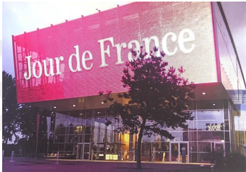
Figure 3.16: T-Mobile Headquarters in Bonn, Germany
