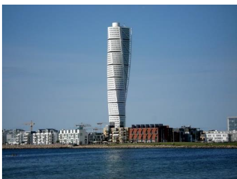
Turning Torso, Malmö, Sweden
