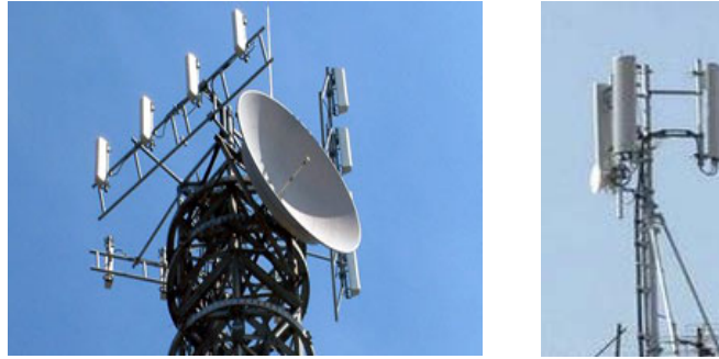
Figure 2.3 - An example of three sector base station antenna types
