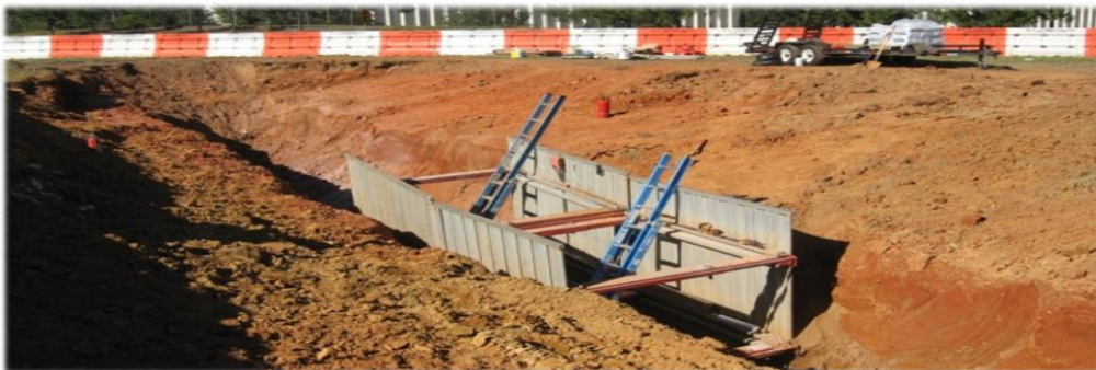
Figure 2.9. Shielded System (Yavaş, 2016)
