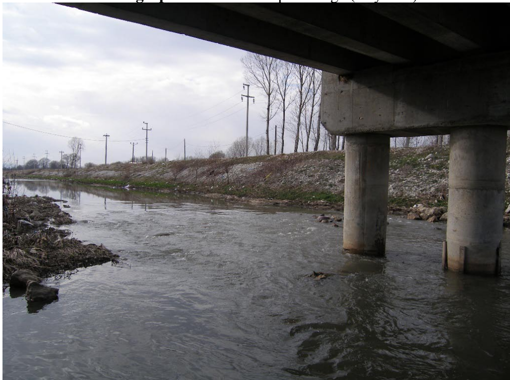
Photograph 10 Station 9 Bridge 8 (Büyüksu)
