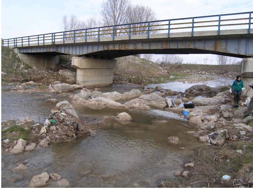
Photograph 9 Station 8 Bolpat Bridge (Büyüksu)
