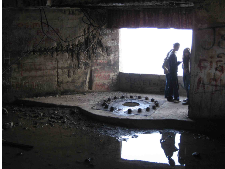
Fig. 2.85 Photograph of the Garipçe fortress, 30 March 2009 (photograph by author).
