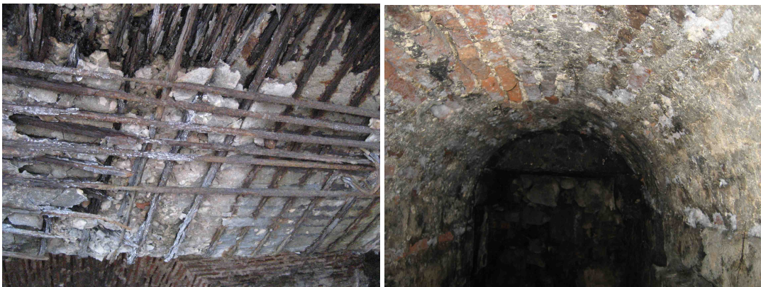
Fig. 4.21 a/b Garipçe fortress underground interior spaces. A view from the exposed ceiling reinforcements on the left and a vaulted chamber on the right with white deposits (probably salt or mold) visible on the bricks (photographs by author).
