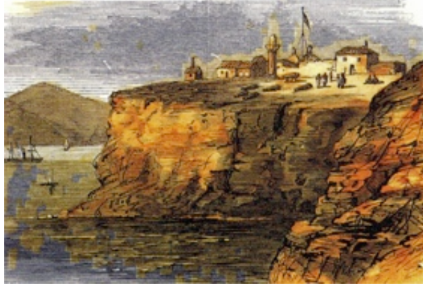
Fig. 2.71 An illustration of the Papazburnu battery from 1877. (From Balcı “Sarıyer”, originally published in L’illustration newspaper, Paris)
