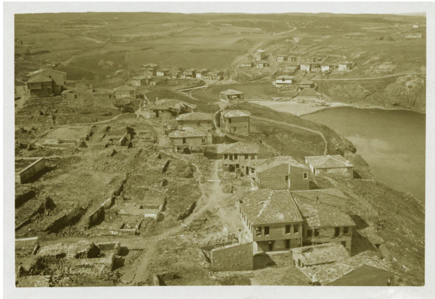
Fig. 2.39 Photograph probably showing the Rumelifeneri village taken from the upper floor of the lighthouse. 74 (Atatürk Library, MTF 1370)
