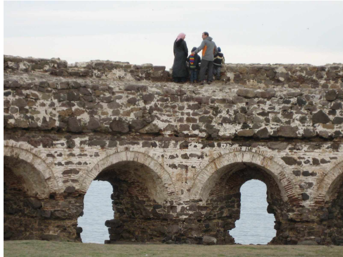
Fig. 4.29 a) A visitor family of four looking out on the sea from the top of the wall-walk at Rumelifeneri fortress (photograph by author).
