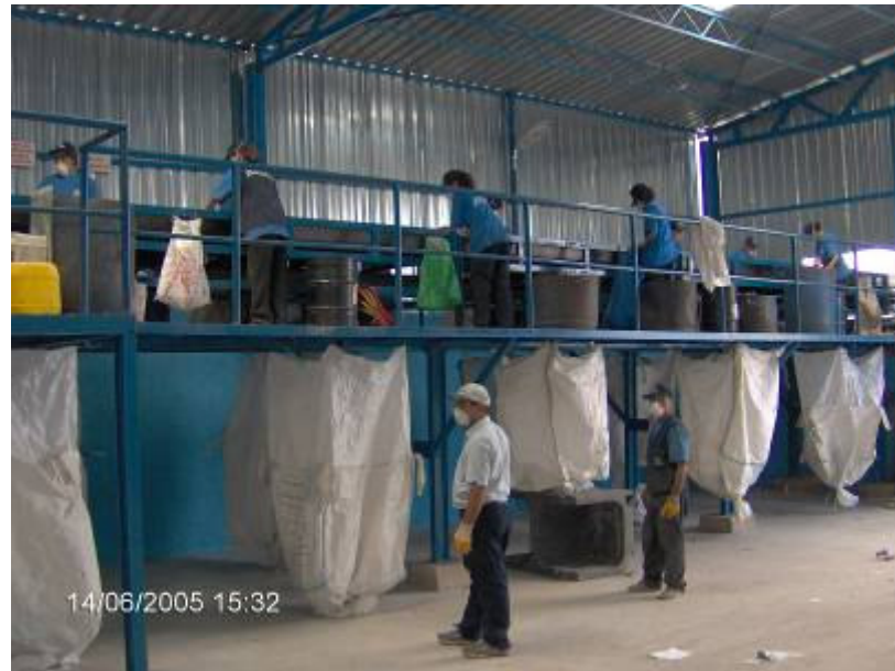
Figure 8.16 The picture of the Sorting Facility in Uzundere Compost Factory, the manual sorting line of the facility
