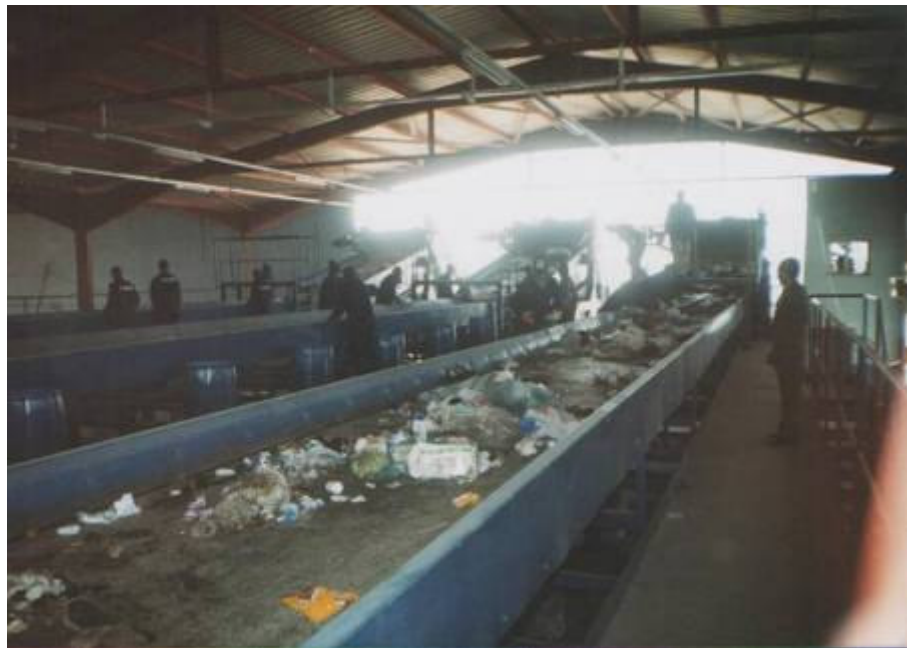
Figure 8.4 The Sorting Facility in Harmandalı Sanitary Landfill
