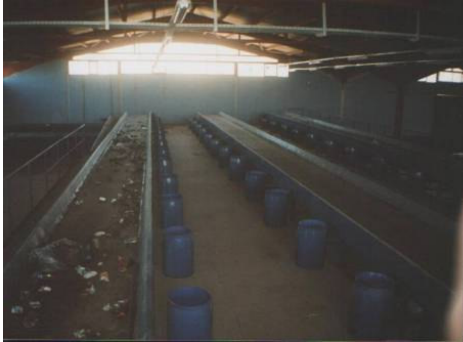
Figure 8.3 The Sorting Facility in Harmandalı Sanitary Landfill
