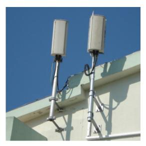
Figure 3.4 Sample wall-mounted RF antennas
