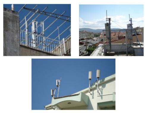
Figure 4.4 Sample roof-top base station installations
