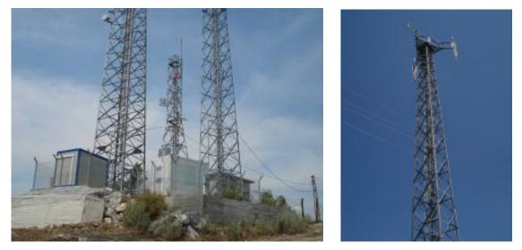
Figure 4.5 Sample green-field (tower) base station installations
