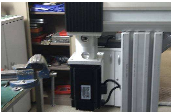
Figure 2.30 Motor connection of source edge silicone mechanism
