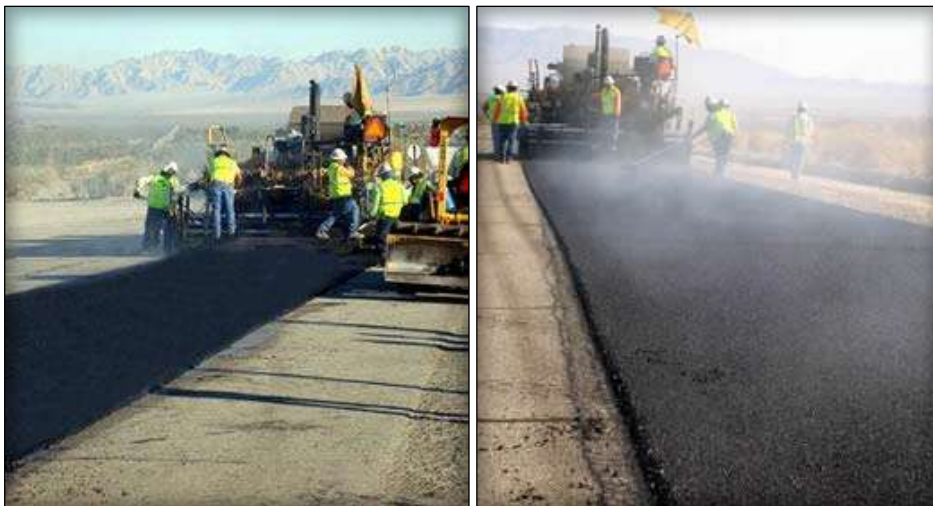
Figure 4.1 Comparison between the warm mix and hot mix asphalt technologies in terms of emission of compaction fumes (Warm mix on the left, hot mix on the right), (Pavement interactive, 2010)
