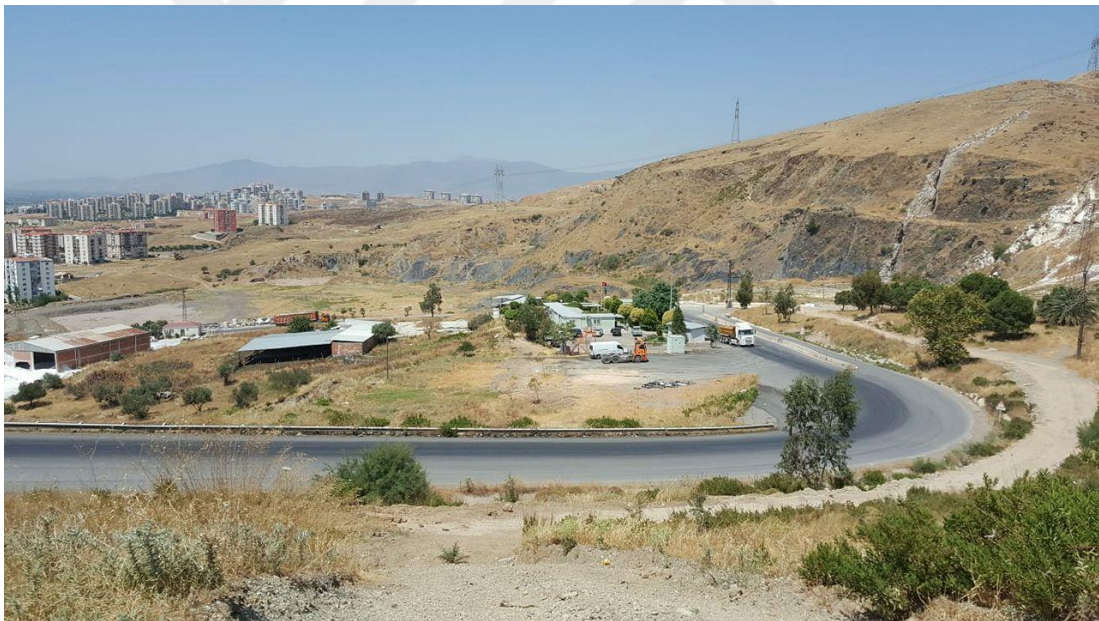
Figure 5.8 The adminastiration buildings in The Harmandalı waste disposal site and landslide direction NW-SE (Personal archive, 2018)
