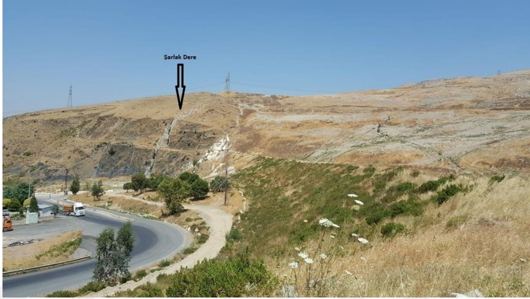
Figure 5.14 Sarlak stream leachate in the Harmandalı waste disposal site (Personal archive, 2018)
