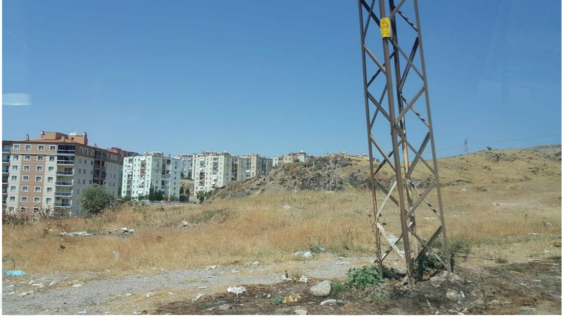
Figure 5.11 The landslide effects in the Harmandalı waste disposal site (Personal archive, 2018)
