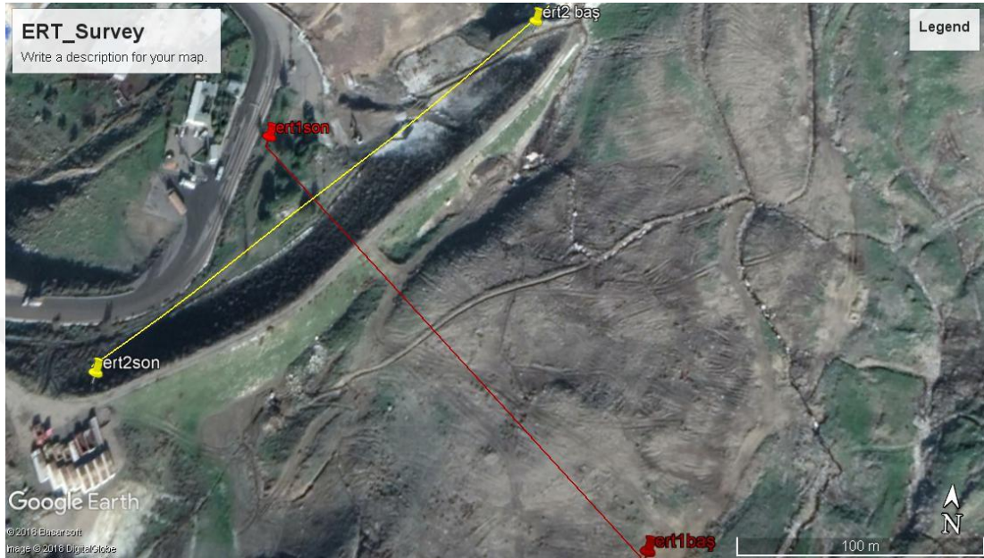
Figure 5.2 Electrical resistivity tomography surveys in Harmandalı waste disposal site (Google Earth, 2018)
