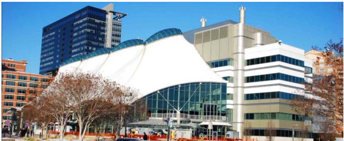
Figure 4.9: Bio-Technology Building on Pier-6
