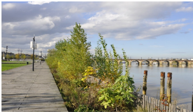
Figure 2.11: Bordeaux Pedestrian Walkway
