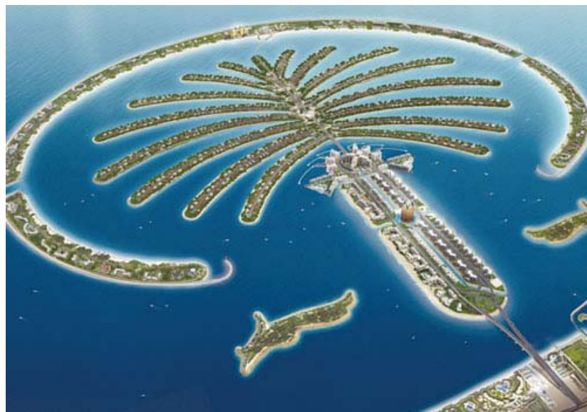
Figure 4.2: The Palm Project, Dubai
