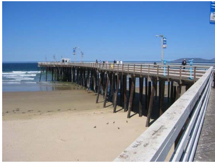
Figure 3.26: Pismo Beach pier, California
