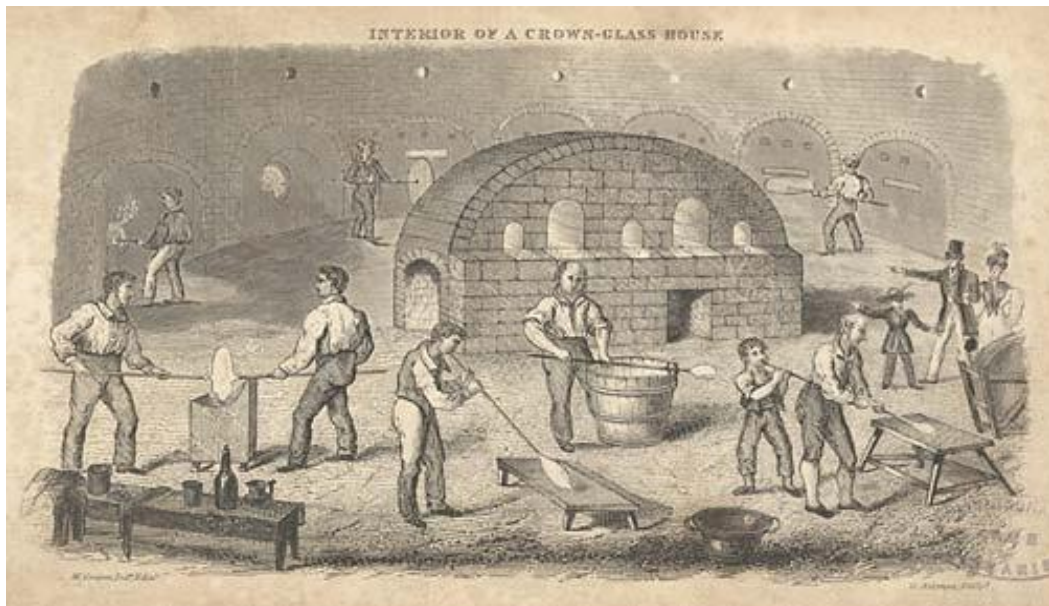
Figure 4.3: The crown glass production
