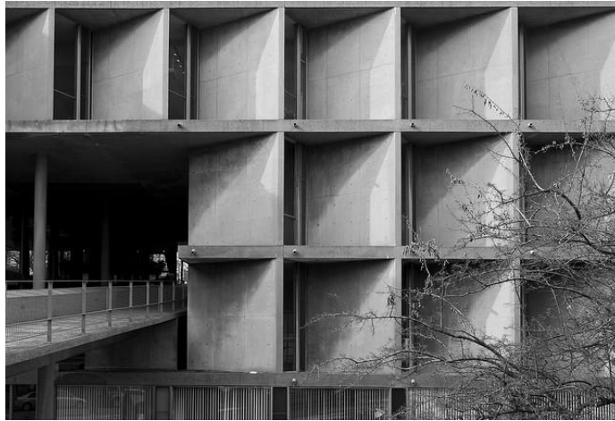
Figure 5.11: The facade of the Carpenter Center
