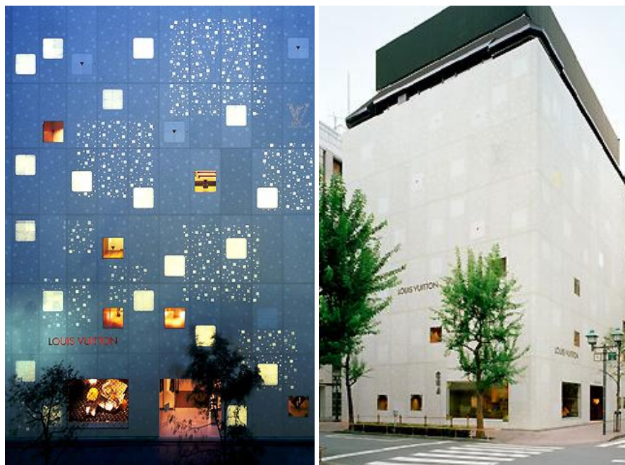
Figure 4.20: White, translucent alabaster is cast in beige glass fiber-reinforced concrete in the skin of the Louis Vuitton flagship store in Ginza, Tokyo
