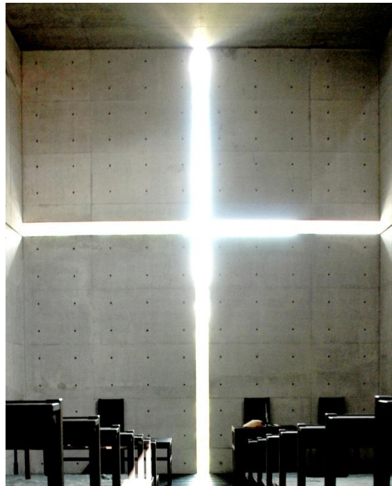
Figure 5.17: The cross cut in the exposed concrete skin
