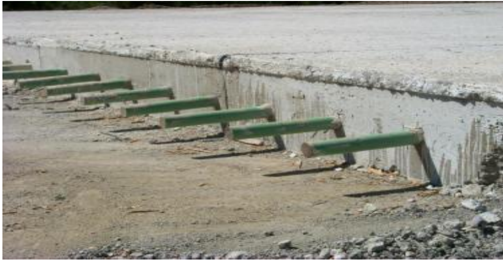
Figure 5.17. Construction joint [70].
