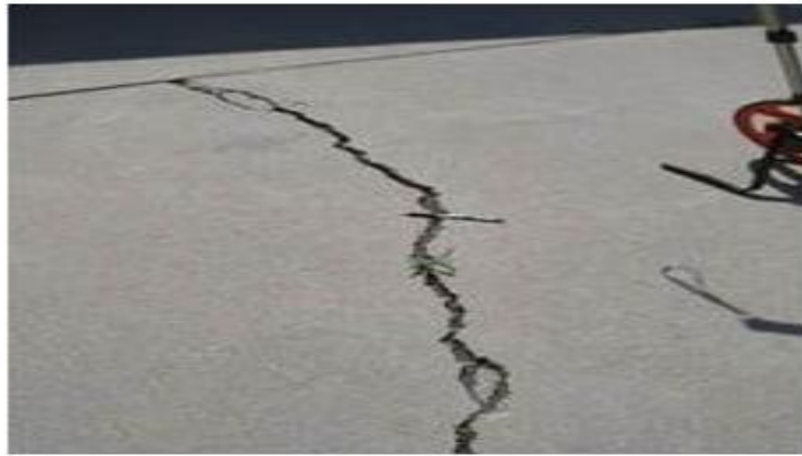
Figure 3.27. Linear cracking [60].
