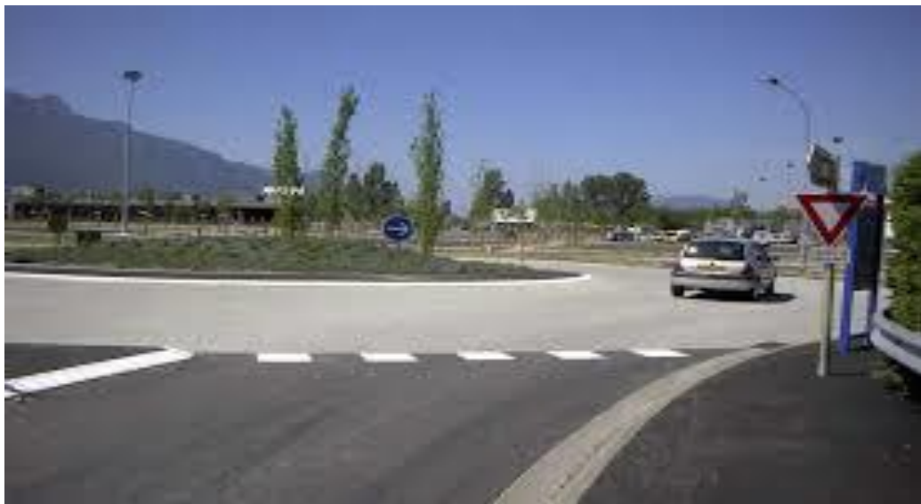
Figure 5.10. Shows the use of rigid paving in the traffic roundabout in French [15].
