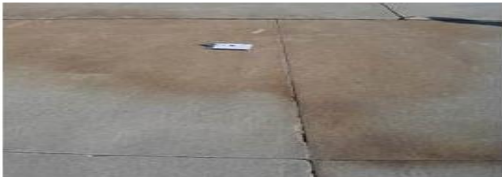
Figure 3.24. Pumping effect [60].
