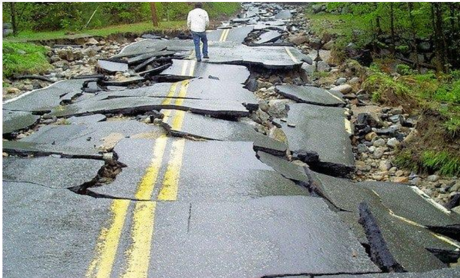
Figure 4.1. Deformation due to environmental factors [42].
