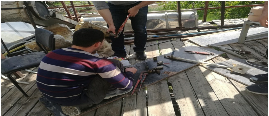
Figure 2. 24 Installs the piping system.
