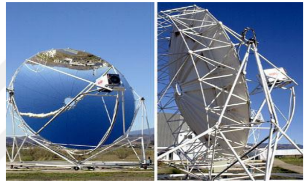
Figure 1. 24 Structure of dish from both sides.
