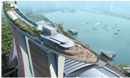
Resim 82: The Marina Bay Sand Hotel, Singapur
