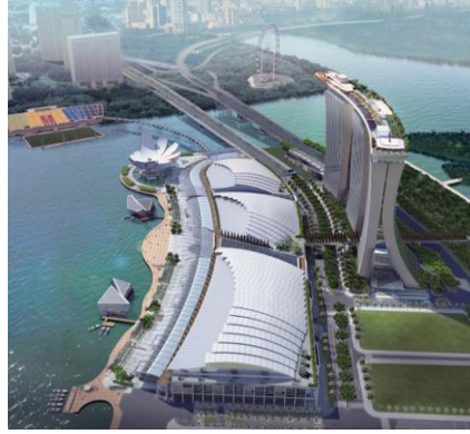
Resim 81: The Marina Bay Sand Hotel, Singapur
