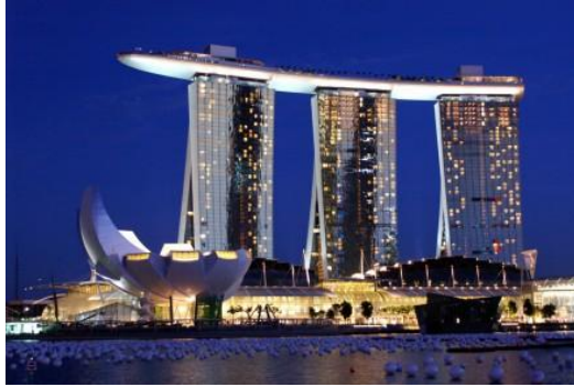
Resim 83: The Marina Bay Sand Hotel, Singapur
