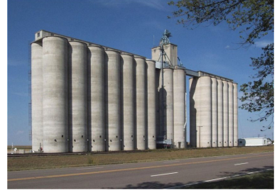
(c) Betonarme Silo
