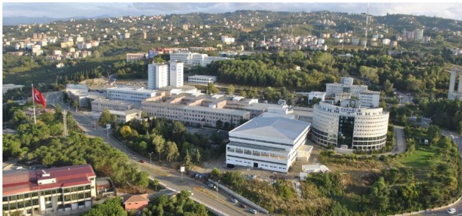
Figure 15. North Farabi Hospital view (URL-17).
