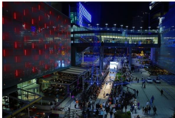
Figure 5.14. Exterior lighting of Armada Shopping Center ( http://www.armadasite.com/armadahayat/galeri )
