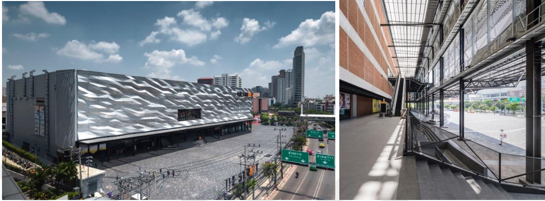
Figure 3.42-3.43: Linear shaped shopping center example, The Street Ratchada, Bangkok, Thailand, 2016
