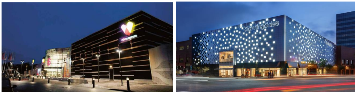
Figure 3.58-3.59: Determined shopping center entrances by lighting http://www.illumni.co/how-to-illuminate-a-shopping-centre-by-eagle-lighting-australia/
