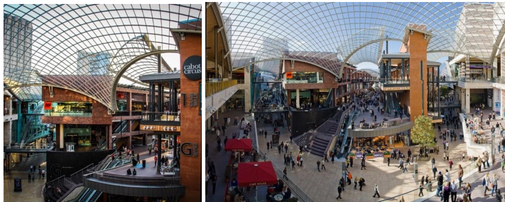
Figure 3.69-3.70: A free-form, shell-shaped glass roof, an award-winning urban regeneration scheme, Cabot Circus shopping center, Bristol, UK, 2008 ( http://www.chapmantaylor.com/projects/cabot-circus )
