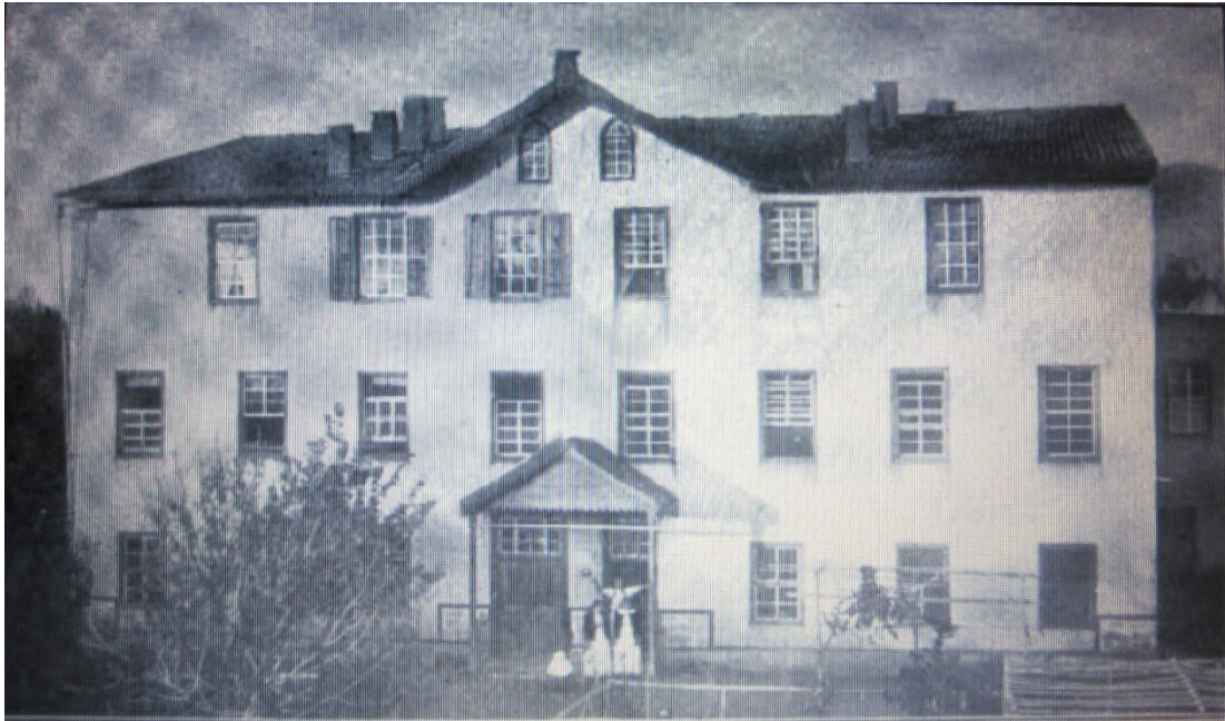
THE HOSPITAL AT VAN
