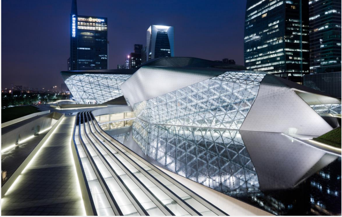
Şekil 5.2.4.1. Guangzhou Opera Binası Kent Silueti, http://www.zaha-hadid.com/architecture/guangzhou-opera-house/
